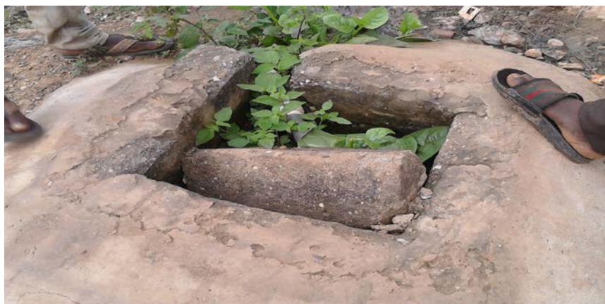
Plate 5. A borehole for groundwater exploitation in Prestea. Source: Fieldwork, June (2014)
