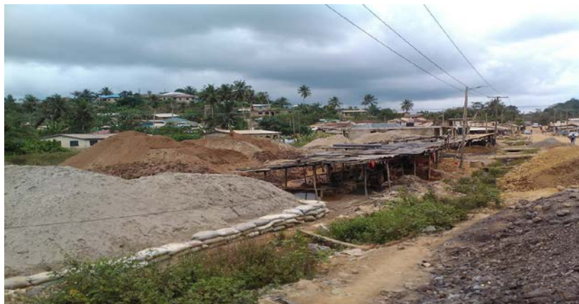
Plate 8. Impacts of land degradation due to illegal small-scale mining activities in Prestea. Source: Fieldwork, June (2014)
