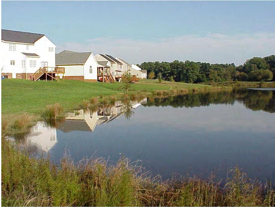
Retention basin – Note flat slopes with “rough” edge and aquatic bench provided as safety and pollutant removal features.
