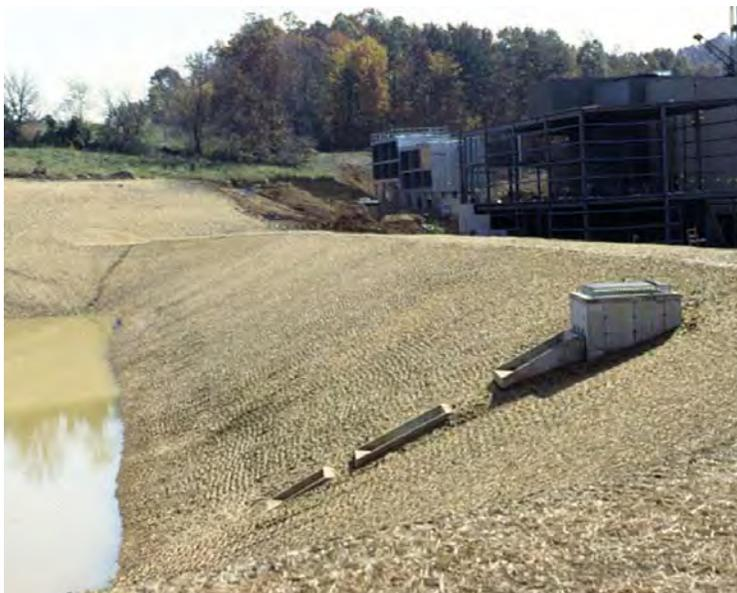
Stabilization of newly constructed Earthen Embankment
