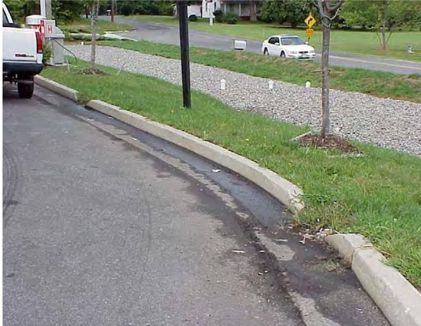
Surface Infiltration Trench. Note grass strip pre-treatment holds heavier particulate pollutants within paved area.
