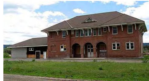
The former Pacific & Idaho Northern Railroad Depot has been awarded several rehabilitation grants and now functions as a community center. (Source: Adams County Historical Society)
