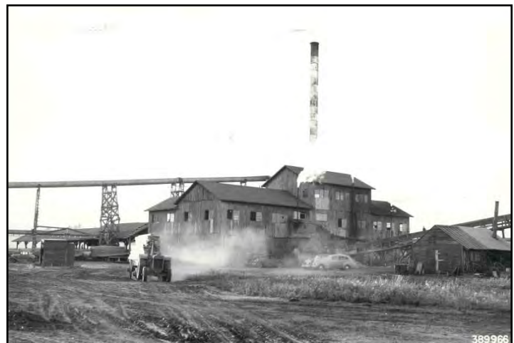
J.P. Dion Mill, Cascade, circa 1924. The mill was largely rebuilt after Boise-Payette Lumber purchased the complex.
