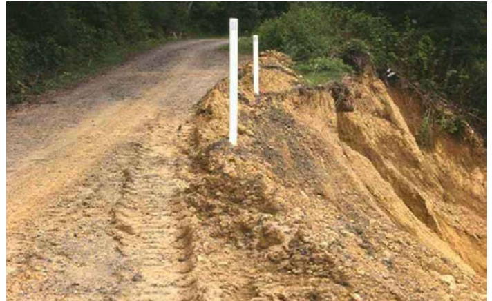
Photo AA. Road related landslide. This fill failure initiated at the point where a culvert discharges to the hillslope.
