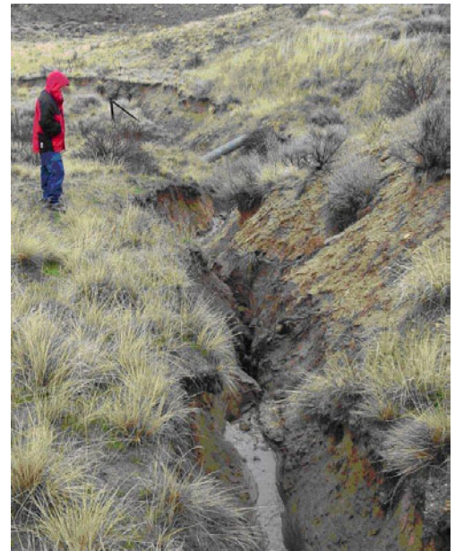
Photo Y. Active gully below culvert due to excessive contributing road length. Note the V-shaped cross section and steep side slopes. This active feature continues over 700 feet to the main valley bottom.
