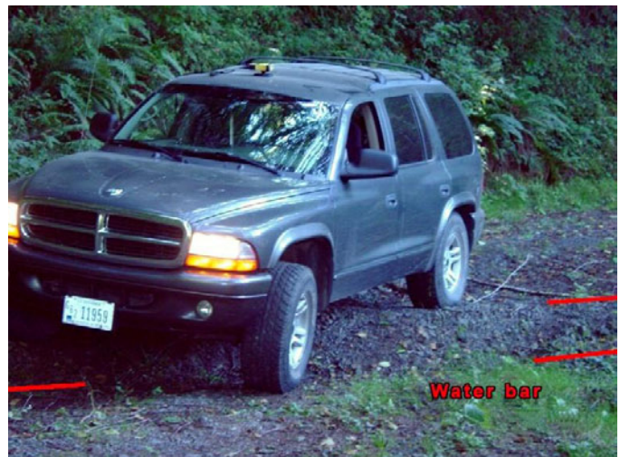
Photo W. Another annotated water bar, with the top and bottom of the water bar marked.
