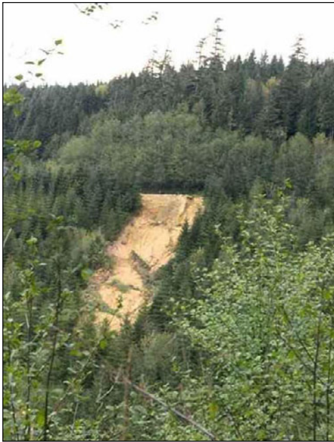
Photo CC-1 and CC-2. These landslides resulted from unstable road fills. Although these are recent events, the gap in vegetation will be notable for many years after the event.
