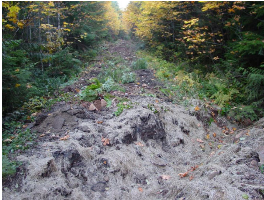
Photo D. Tilled road with water bar.
