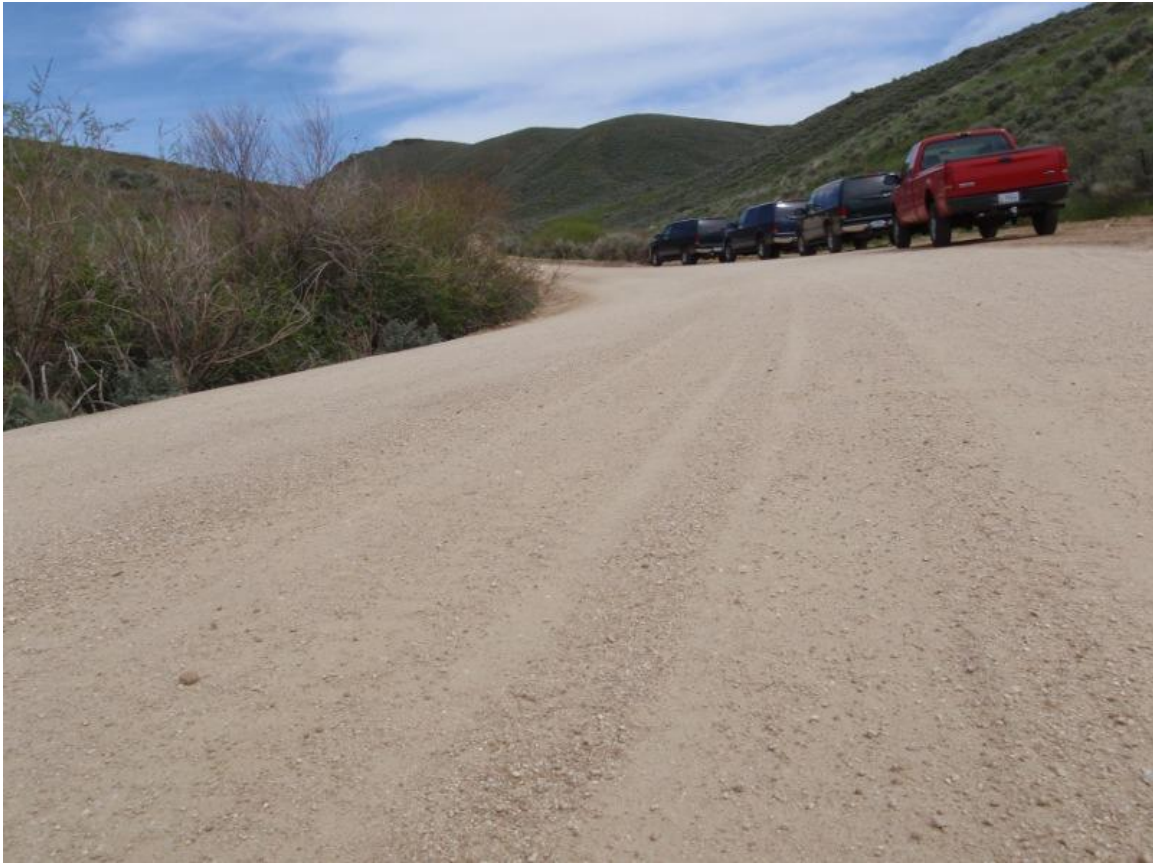
Photo K. This outsloped section of road drains diffusely. Note that the photo is level and the surface of the road is outsloped.
