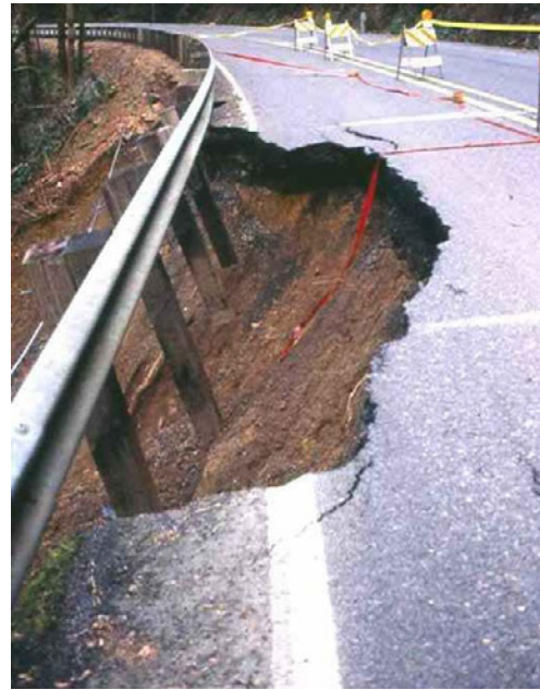
Photo CC-1 and CC-2. These landslides resulted from unstable road fills. Although these are recent events, the gap in vegetation will be notable for many years after the event.
