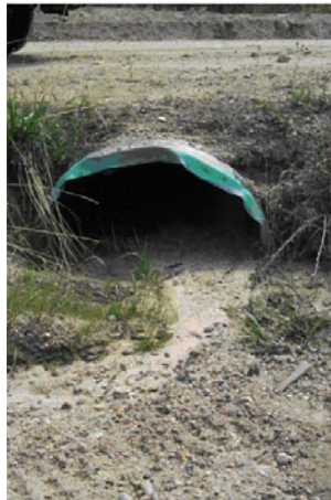
Photo L. Steel 18" culvert inlet, 20-80% occluded by sediment. Note that there is some crushing, but this is not significant because it does not cause any problems, and occlusion is the main issue here.
