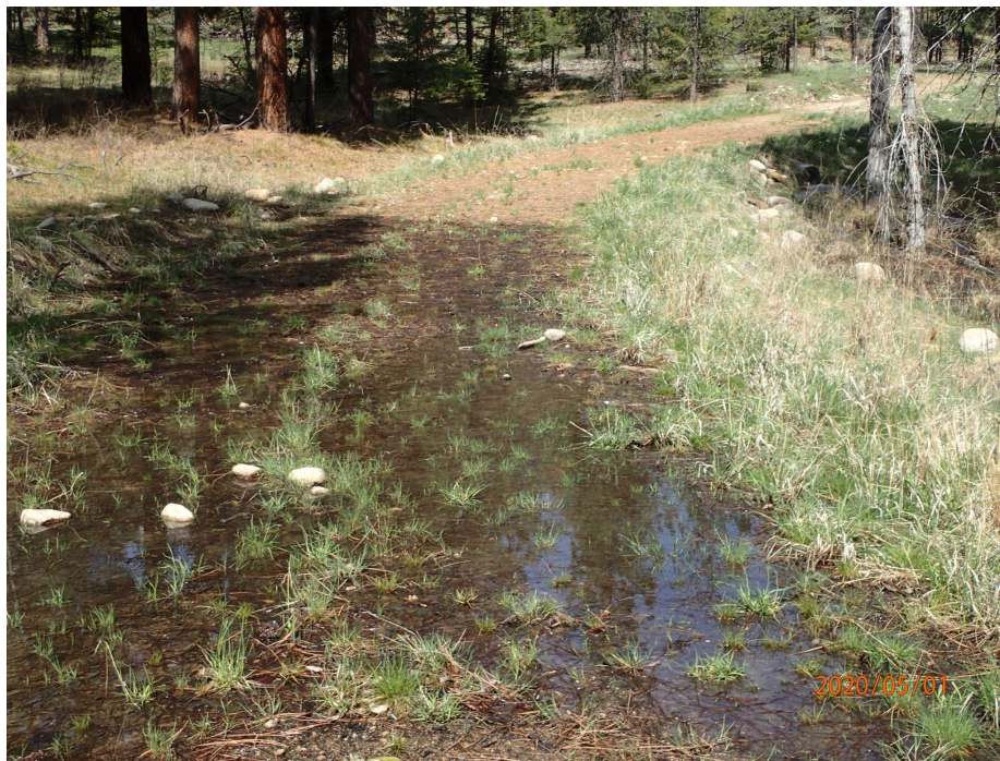
Figure 9. Inadequate drainage on newly constructed Westside project road.
