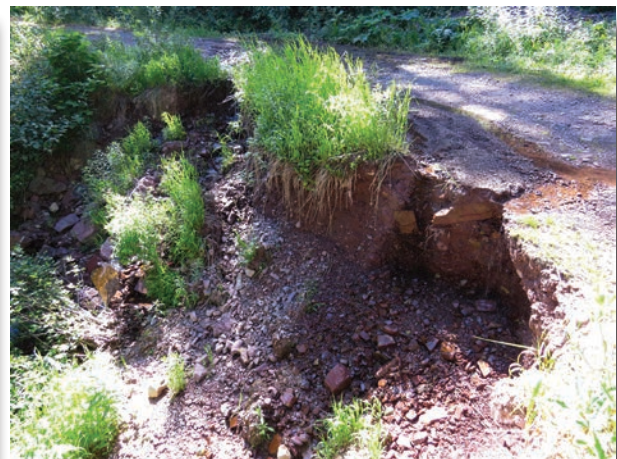
Road 1673 looking downstream at road-fill erosion.
