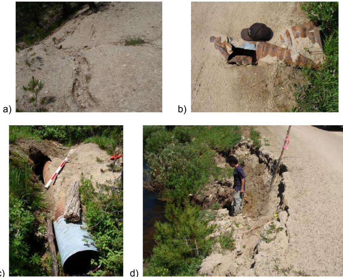
**Photo 4.** Examples of drain point condition problems including: a) erosion at a broad based dip, b) a rusted and damaged ditch relief culvert, c) a stream crossing with flow around and possibly over the pipe, and d) a non-engineered feature where the stream is cutting into the road fill material.
