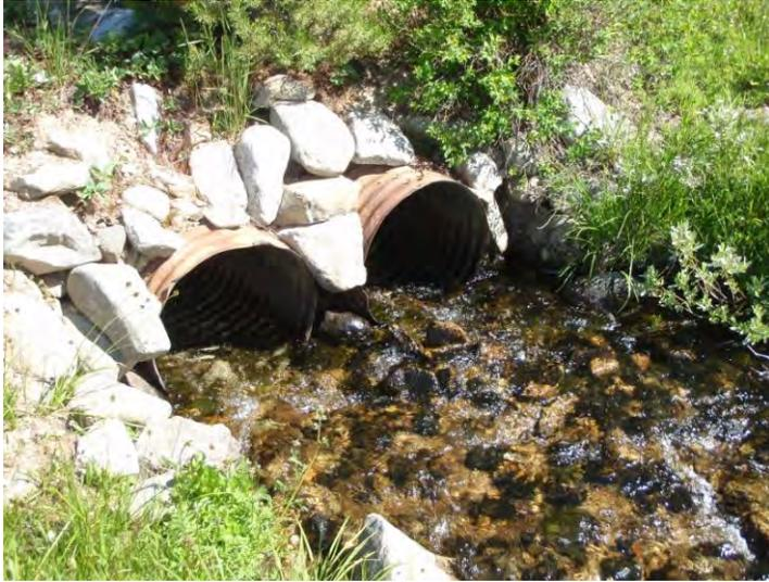
**Photo 5.** Many stream crossings such as this one have more than one pipe to prevent blockage or flow diversion. SBI figures do not account for the presence of multiple pipes which means some SBIs may predict higher risk than what actually exists.
