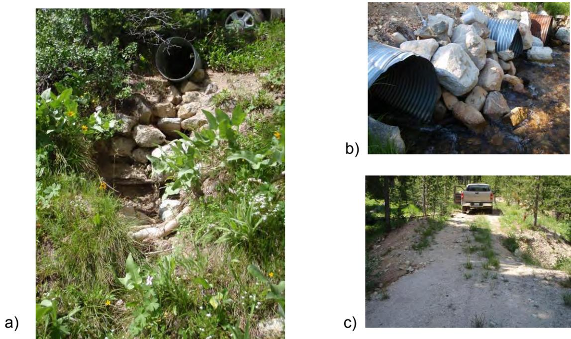
**Photo 2.** Photos of high delivery drain points. a) Gully at outlet of highest delivering drain point in the entire basin, located on NFSR 569. b) Sack Creek stream crossing on FR 582, one of top 24 highest delivering drain points in basin. c) Eroded and dilapidated stream crossing of Bearskin Creek on NFSR 563C1.
