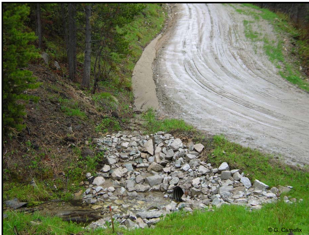
Photograph 1. An example of an ineffective Best Management Practice (BMP) that failed to significantly reduce major impacts of land use on aquatic systems on the Bitterroot National Forest, MT. High levels of fine sediment from road impacts continue to be funneled directly to this stream via road drainage features, despite the recent addition of rock to the stream crossing in 2005. The stream is in the East Fork of the Bitterroot River watershed, which is designated as having impaired water quality due to sedimentation. This watershed provides habitat for bull trout, listed as threatened under the Endangered Species Act, and imperiled western cutthroat trout. Increases in fine sediment significantly reduce the survival of both these native trout, as discussed in the text. Photograph: G. Carnefix.
