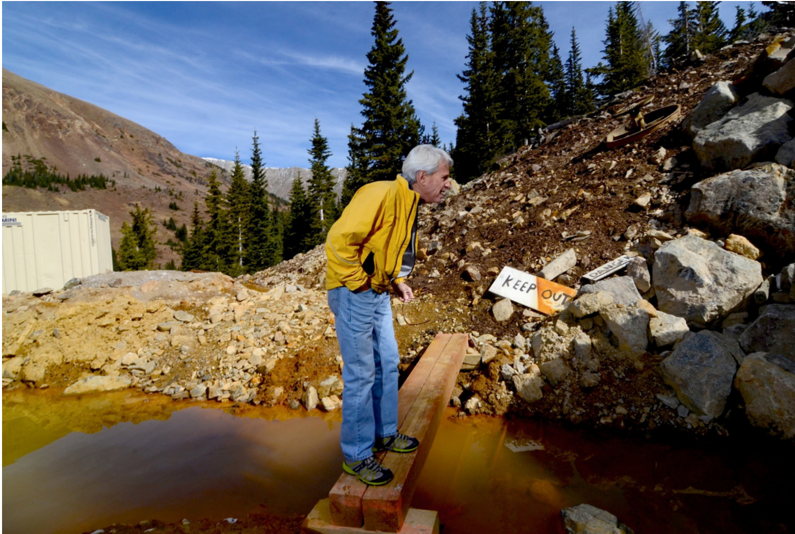
Gary Martinez peers into a tunnel at Pennsylvania Mine that was officially plugged in 2014. An 18-foot-thick bulkhead of steel-reinforced concrete will help reduce the amount of heavy metals, such as zinc, that drain into Peru Creek and upper sections of the Snake River. Researchers have found that the area still contains high levels of rare earth metals.
