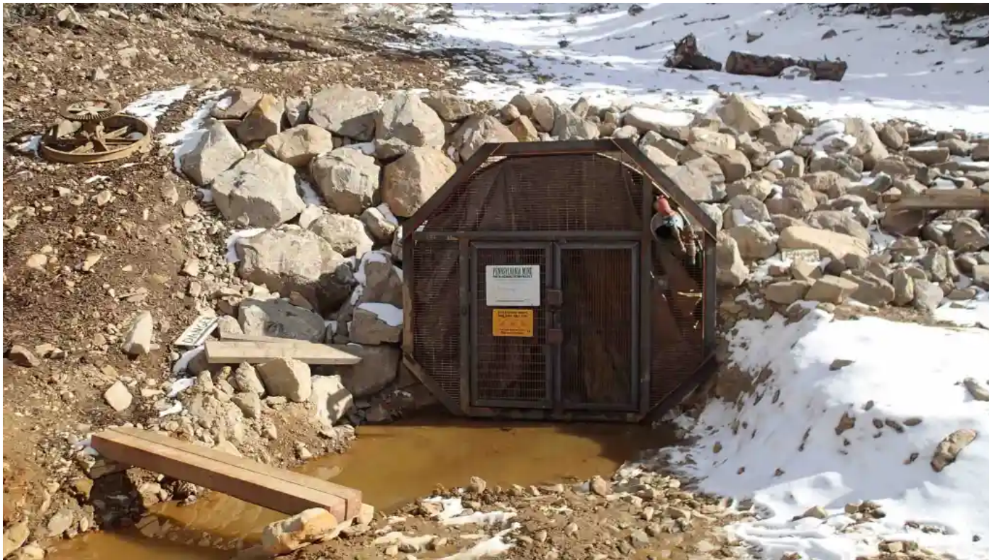
Portal of the Pennsylvania Mine in Summit County, upstream from Keystone Resort. Photo courtesy of Jeff Graves, Colorado Division of Reclamation, Mining and Safety
