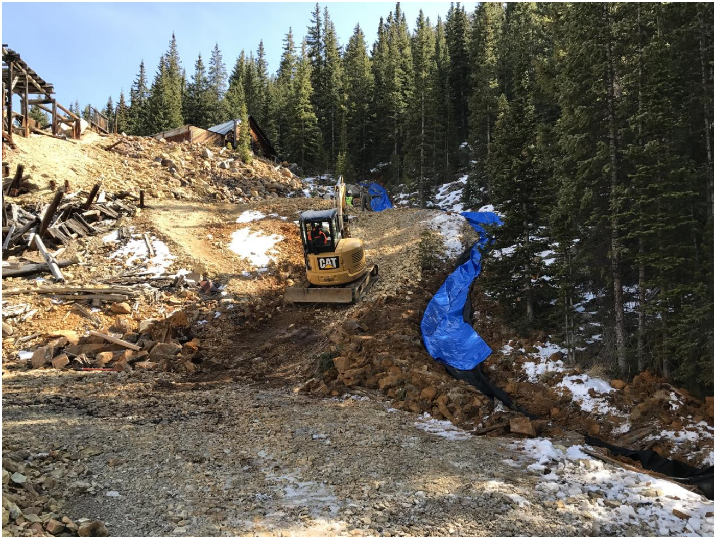
Jumbo Mine looking up at channel liner installation from lower middle section of waste rock pile. Photo credit Environmental Protection Agency.
