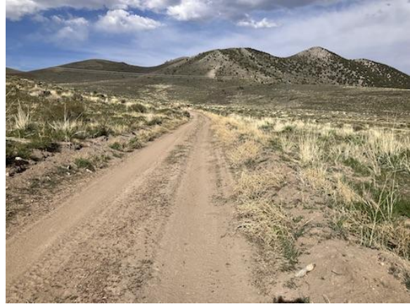
42758 after being graded
