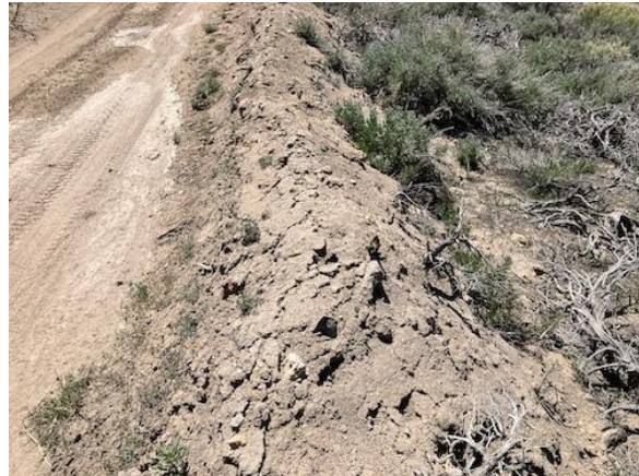
Road 22536 after grading
