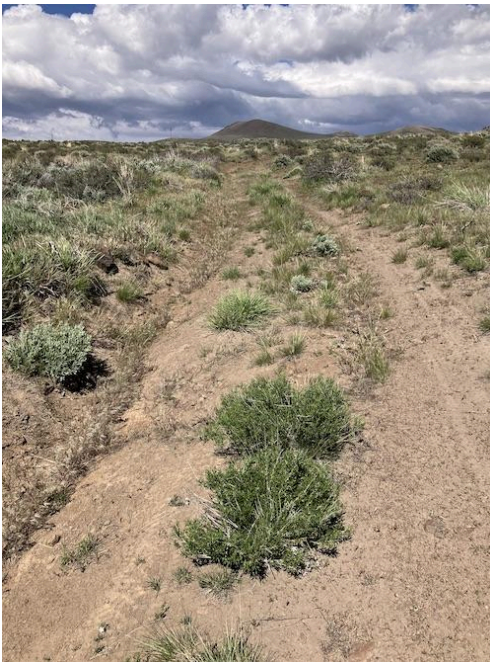
Road now in 2026—9' wide, eroded on slopes, less so on level ground.
