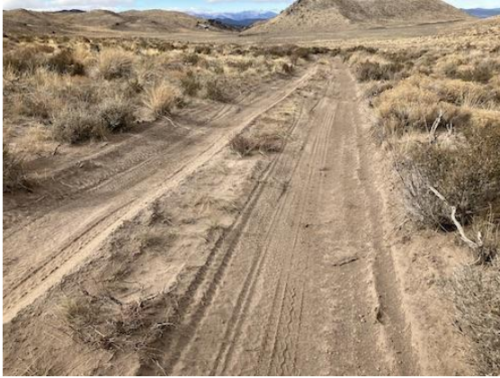
Damage done by the water truck traffic.
