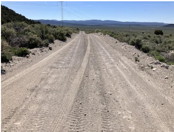
Looking south from Laydown Area 1 on 42754
