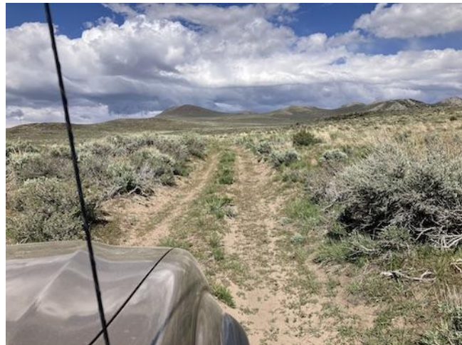
Road now in 2026—9' wide, eroded on slopes, less so on level ground.
