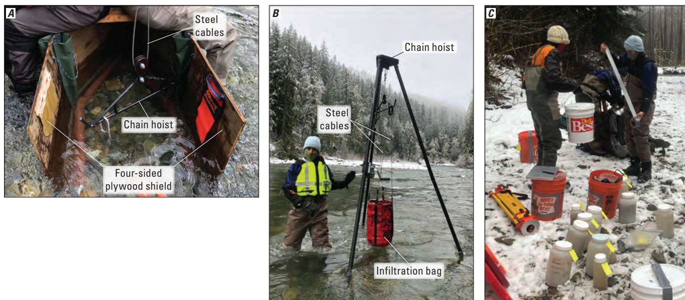
Figure 5. A four-sided plywood shield is installed immediately upstream from buried infiltration bag and chain hoist centered over buried infiltration bag (A), the infiltration bag hanging from chain hoist (B), and all material in the infiltration bag, including water and sediment, is packaged in on-site containers (C), upper Sauk River study site, March 2021.
