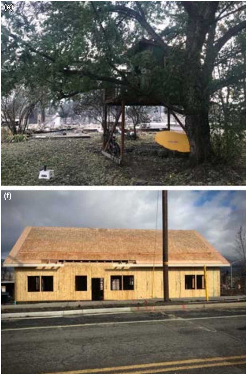
FIGURE 10.1 Two views (a, b) of mobile homes destroyed by the Almeda fire; (c) a fire-prepared church untouched by flame; (d) unusual creek-side surviving house with dense vegetation; (e) interesting surviving treehouse (notice the burned-out structures right next to it); and (f) postfire reconstruction with flammable wood (no home hardening). All photos, D. DellaSala.
