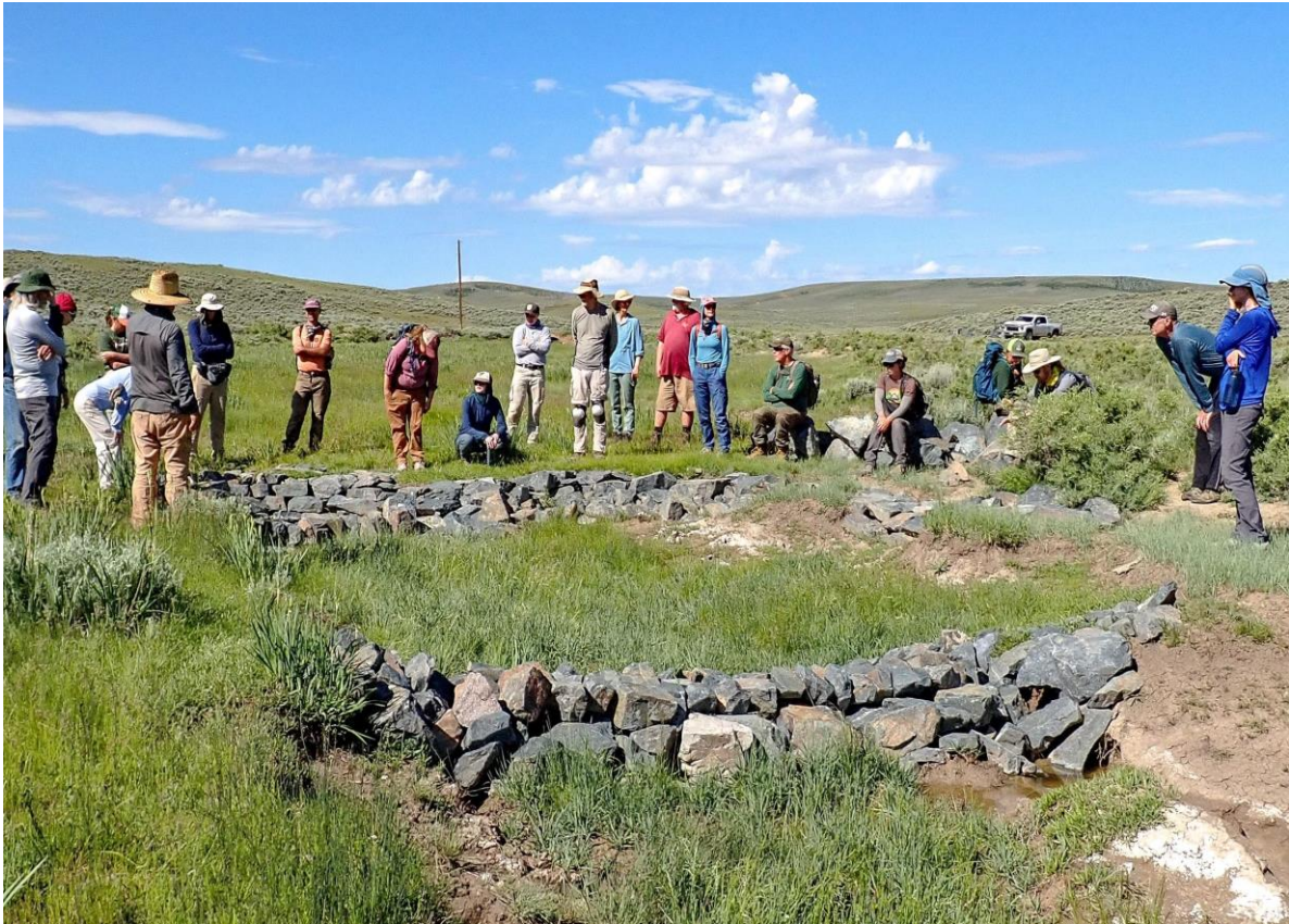
Figure 2 • Low-tech “geoengineering.” A group of restoration volunteers examine their work three years after the installation of structures designed for erosion control, rewetting of grassland meadows, and reestablishing the flood plain on sites that were previously being drained and converted to sagebrush. Photo by Cathy Tate.
