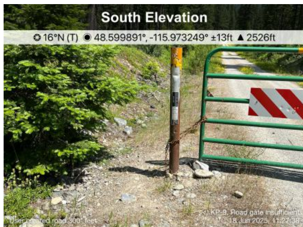
Gate bypassable, left.
