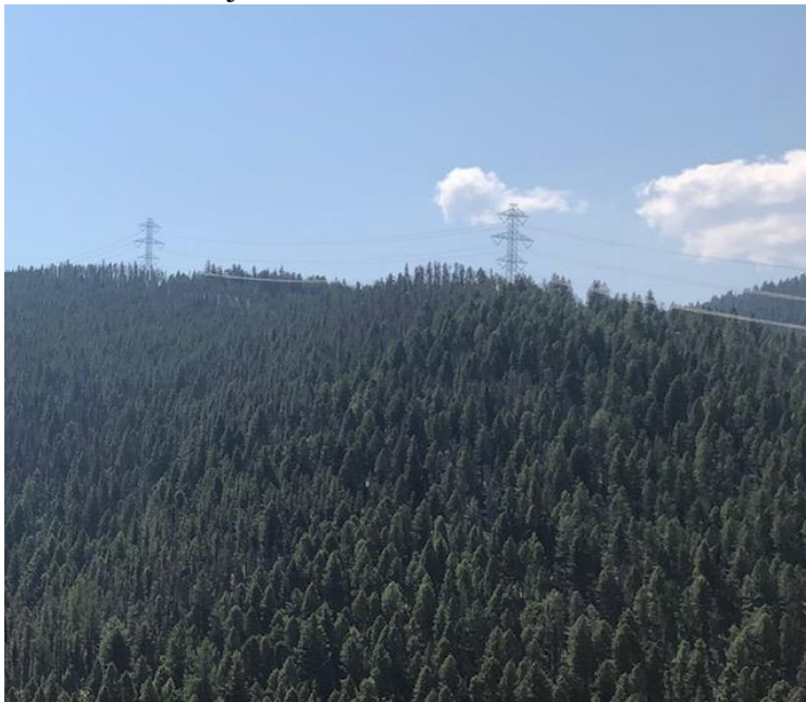
Powerline in Project area under dense fuels.
