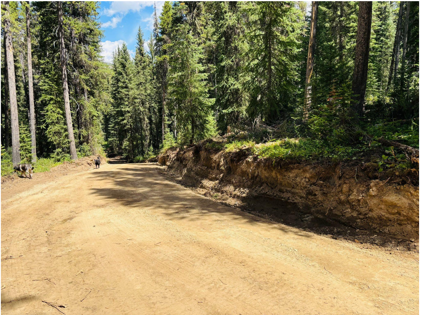
Widening of road to upper Woody Creek Bridge
