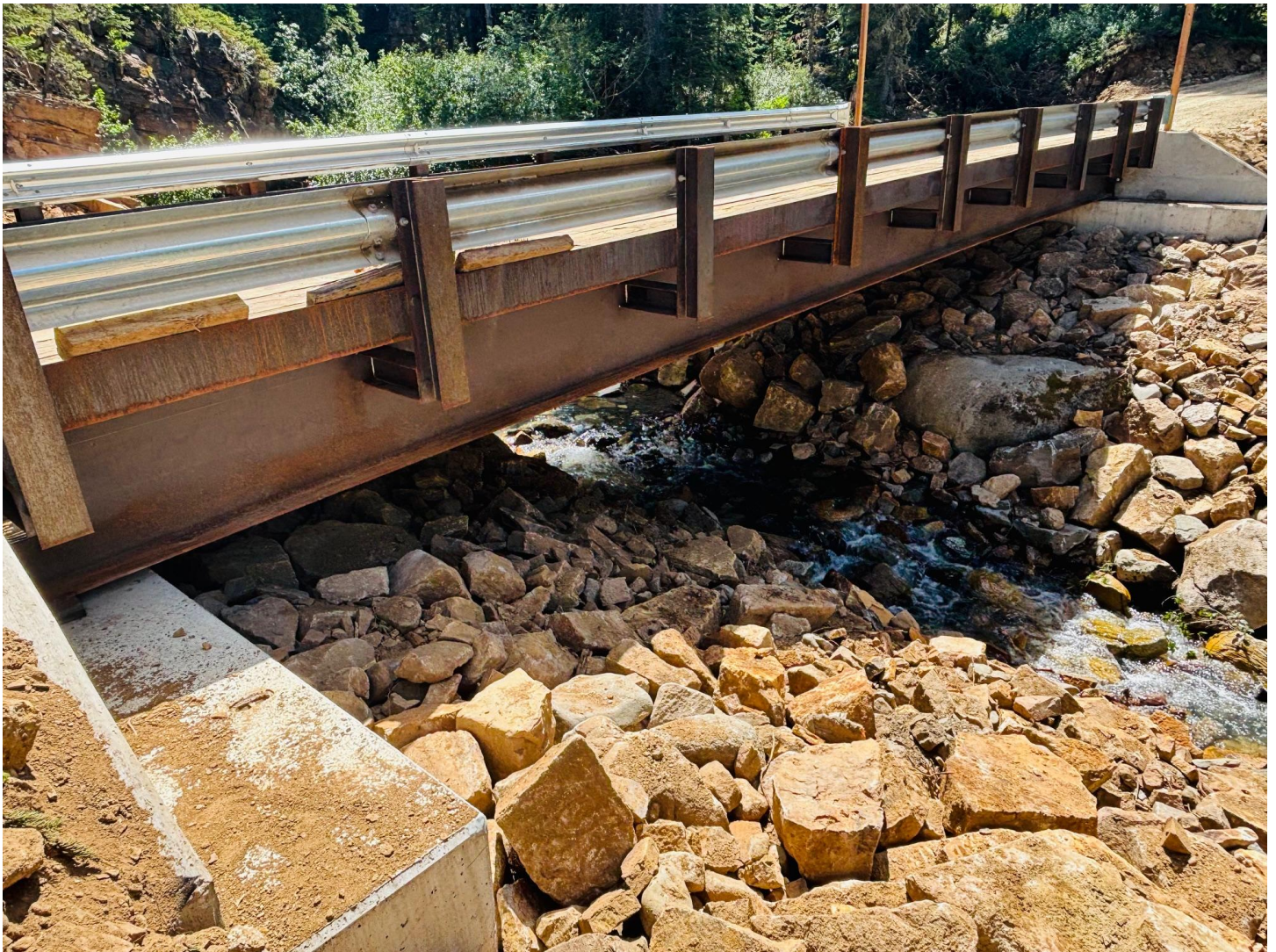
Upper Woody Creek Bridge completed July 2025
