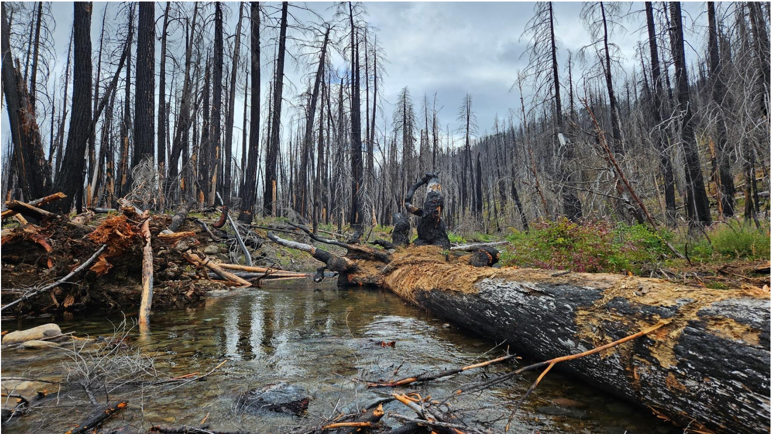
Cub Creek Phase II Post-Project Photo Point 2 (looking upstream): alluvium (fill) and large wood was added to the channel during Phase II.
