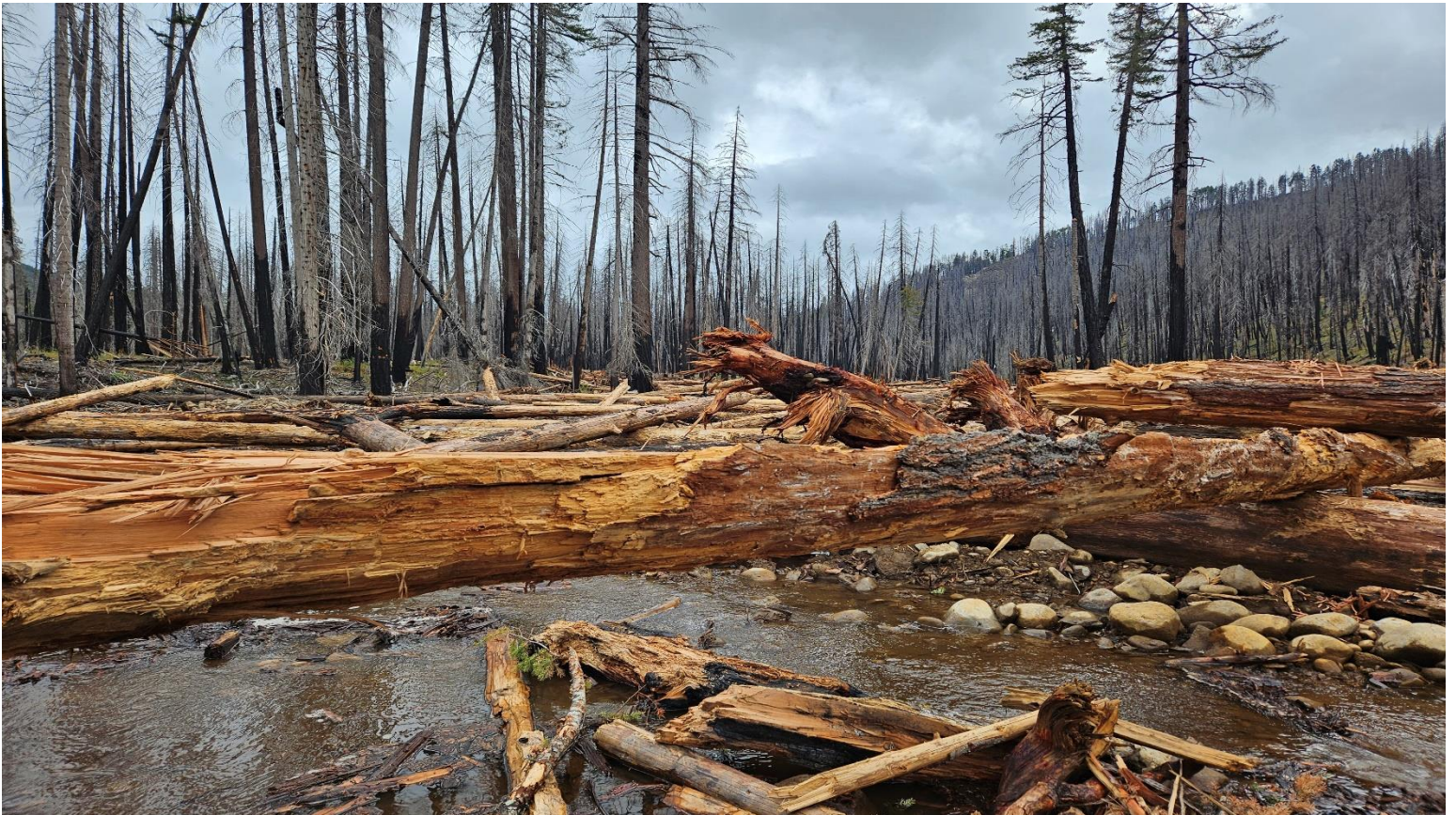
Cub Creek Phase II Post-Project Photo Point 5 (looking south): alluvium was removed (cut) from this area, redistributed to the main channel to match elevations, and large wood was added during Phase II.
