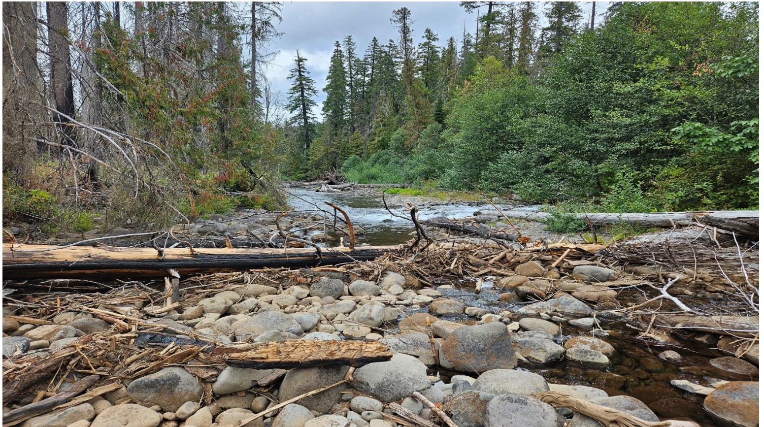
Cub Creek Phase II Post-Project Photo Point 8 (looking downstream): alluvium (fill) and large wood was added to the channel during Phase II.
