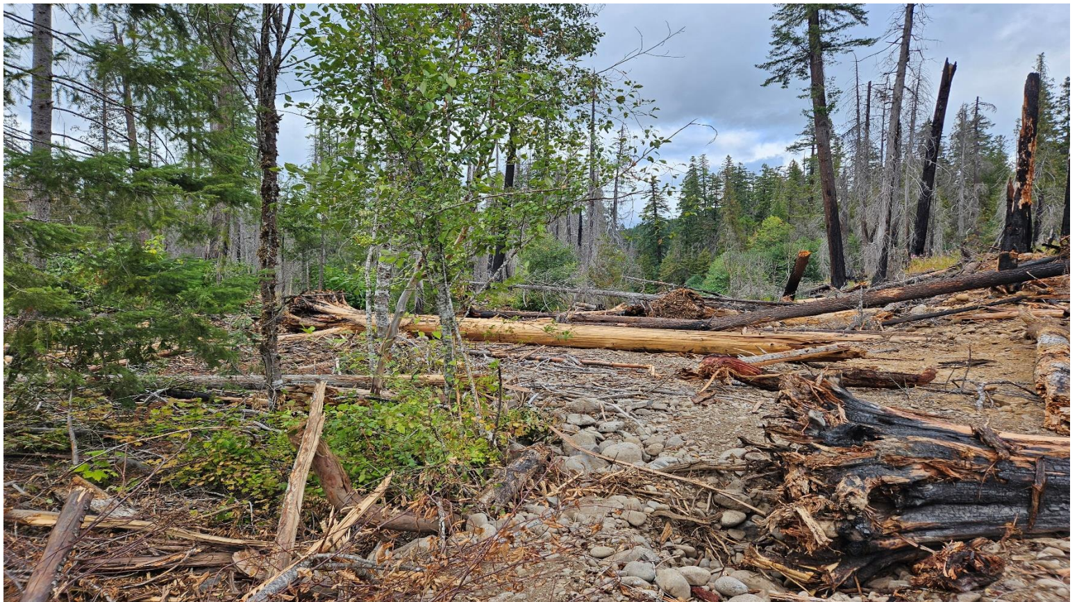
Cub Creek Phase II Post-Project Photo Point 7 (looking downstream): alluvium (fill) and large wood was added to the channel during Phase II. The floodplain was dry when photopoints were taken, but was wet on October 01, 2024.
