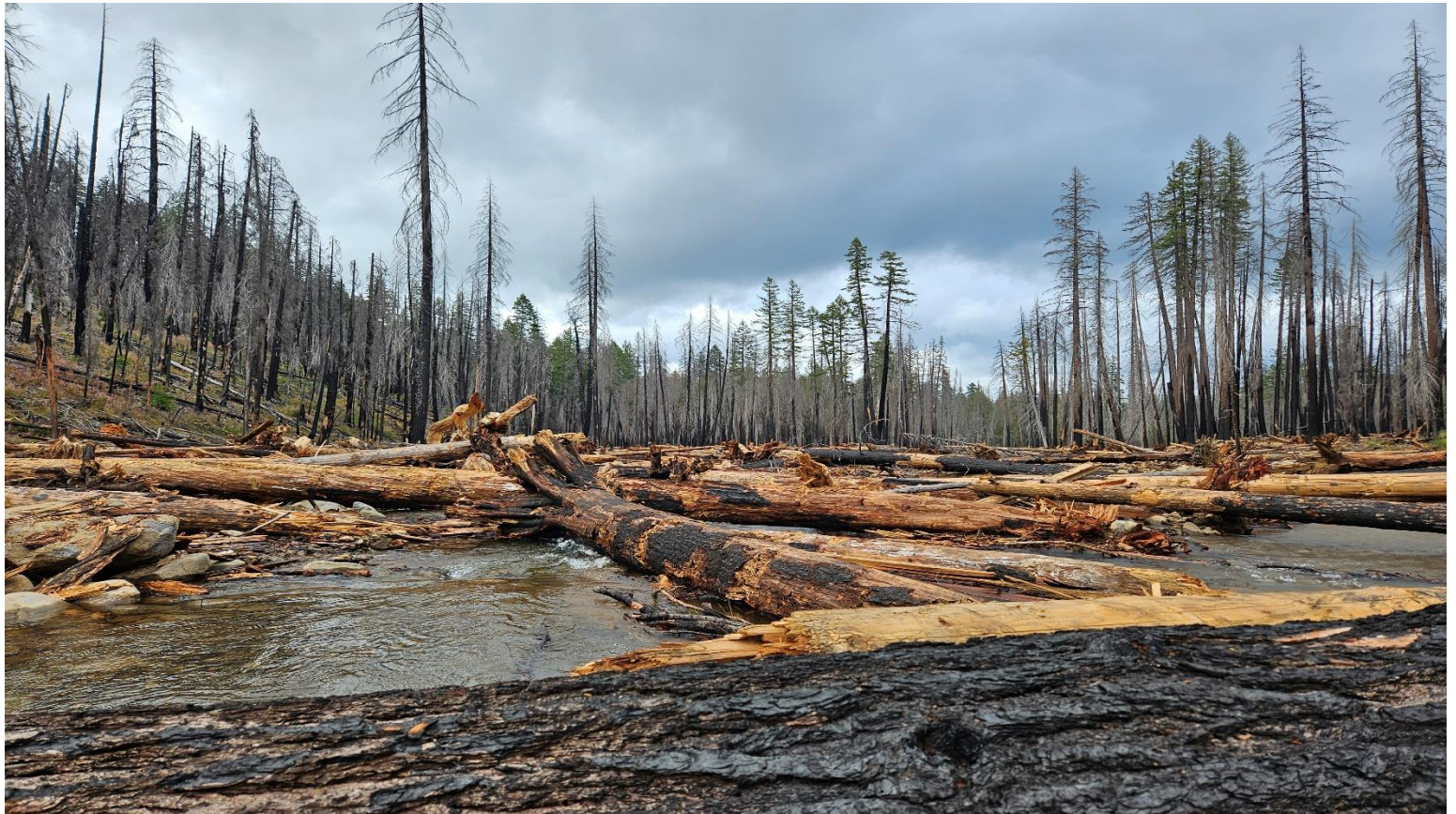
Cub Creek Phase II Post-Project Photo Point 3 (looking downstream): alluvium (fill) and large wood was added to the channel during Phase II.
