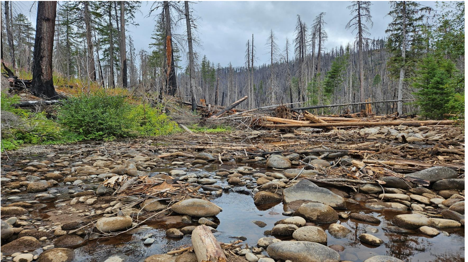
Cub Creek Phase II Post-Project Photo Point 8 (looking upstream): alluvium (fill) and large wood was added to the channel during Phase II.
