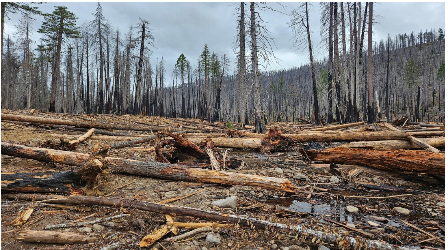
Cub Creek Phase II Post-Project Photo Point 7 (looking upstream): alluvium (fill) and large wood was added to the channel during Phase II.
