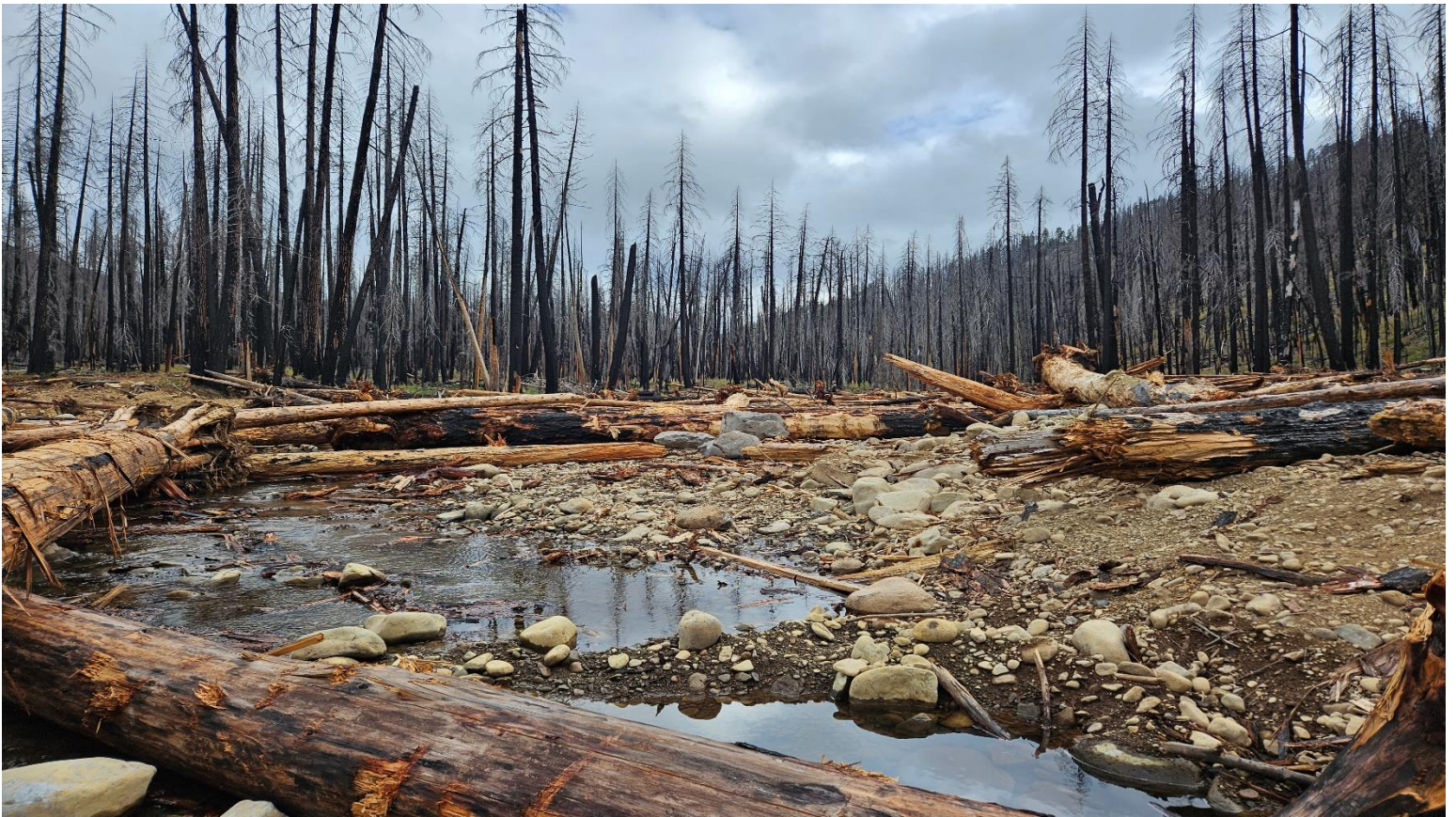
Cub Creek Phase II Post-Project Photo Point 4 (looking south): alluvium was removed (cut) from this area, redistributed to the main channel to match elevations, and large wood was added during Phase II.
