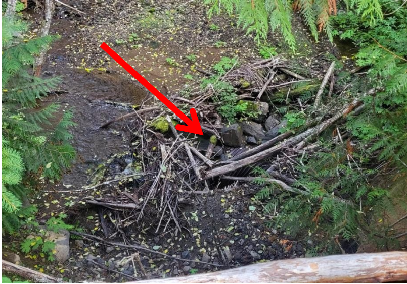
Plugged inlet at South Fork Swampy Creek. Arrow is pointed at inlet.
