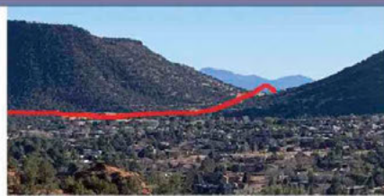
Location just south of the VOC where APS wants to build an above ground high-voltage power transmission line.
