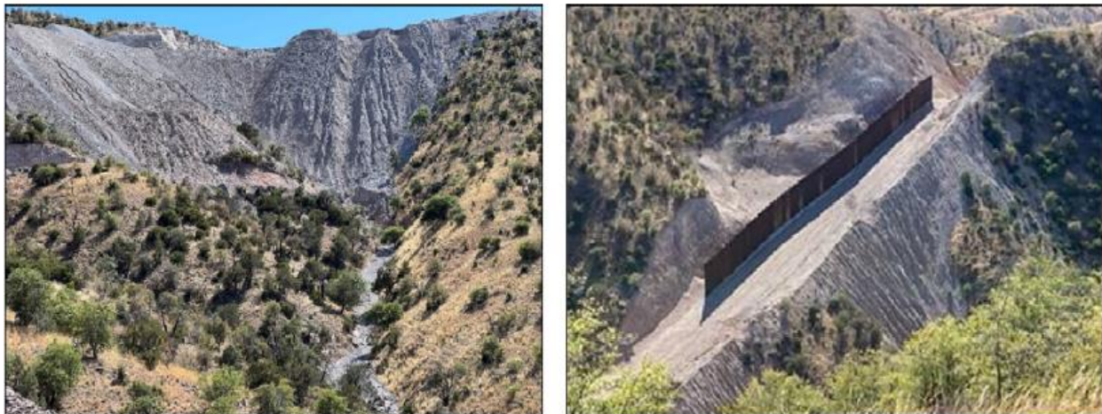
Erosion below the site of a cleared staging area (left); erosion below an area where only several border barrier panels were installed as of January 2021 (right).
