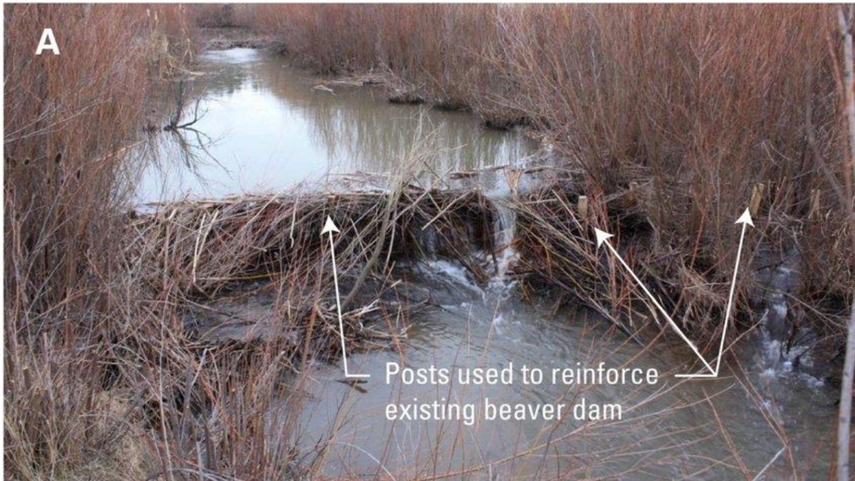
Figure C4. Examples of untreated wooden posts being used to support an existing beaver dam so that it can last through high-water events (Wheaton et al. 2019).
