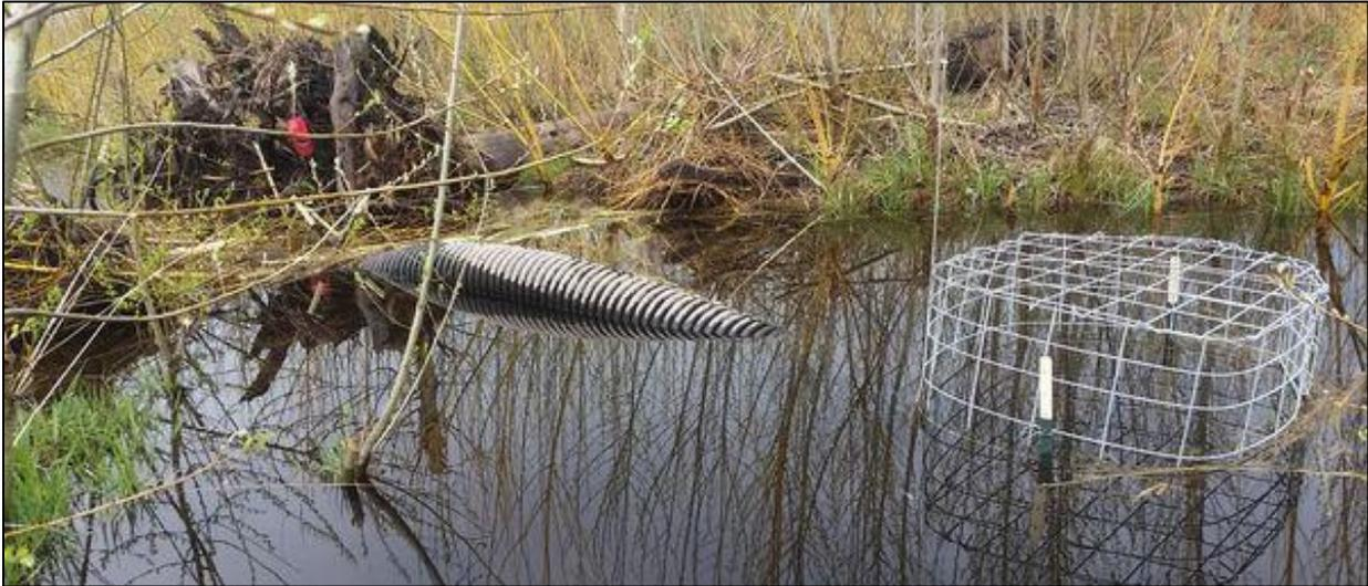
Figure A6. Installed view of the flexible pond leveler device for controlling beaver-flooding issues. The beaver dam is notched to lower the pond water level to the point that is tolerable for the situation, then a flexible pipe is run through that notch in the dam. Photo by Elissa Chott.
