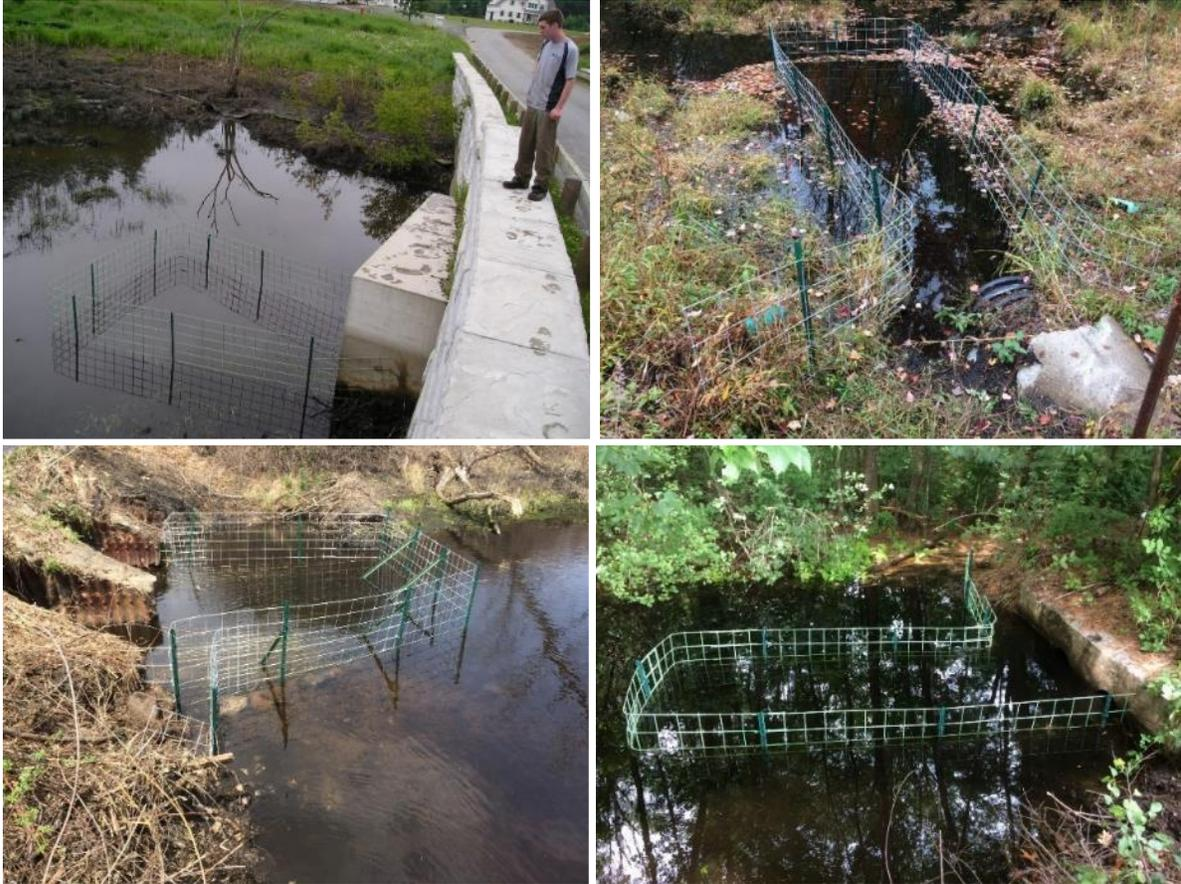
Figure A4. Examples of various types and shapes of fences used to keep beavers from plugging man-made pinch-points like culverts, bridge gaps, and headgates. Photos supplied by Google Images.
