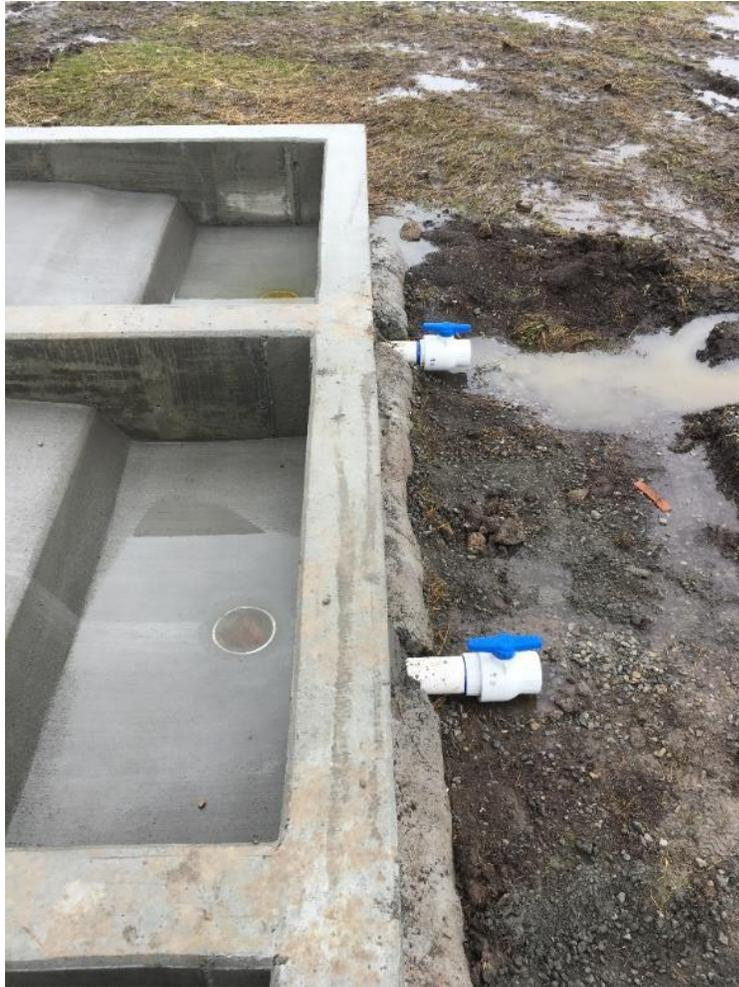
Figure E4. Concrete pads designed specifically for beaver holding facilities. The pads are poured to provide a swimming trough at the back end of the caged area and includes a gentle slope into the swimming area for beavers to easily climb in and out. Drainpipes are fitted into the structure to allow for easy draining and cleaning of the holding facilities between beaver cohorts.
