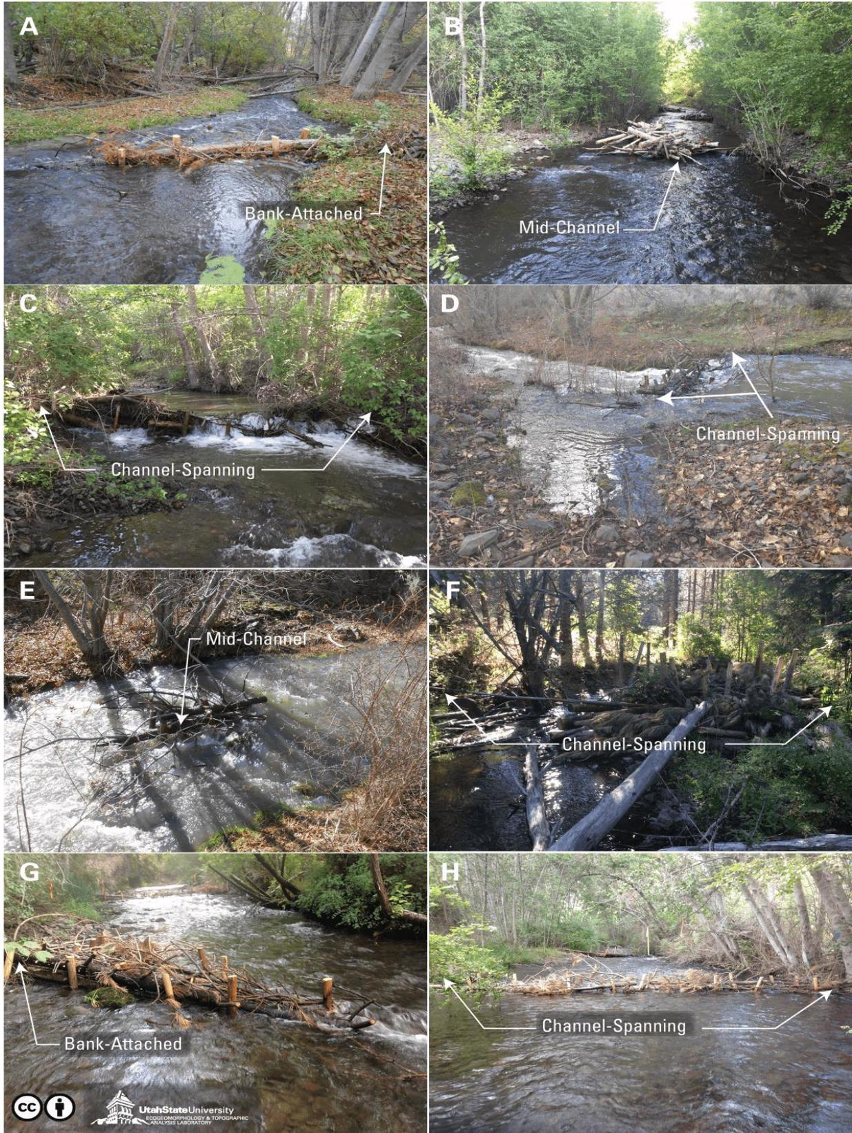
Figure C5. Examples of the various forms and functions of Post-assisted Log Structures (PALs). Figure from Shahverdian et al. (2019).
