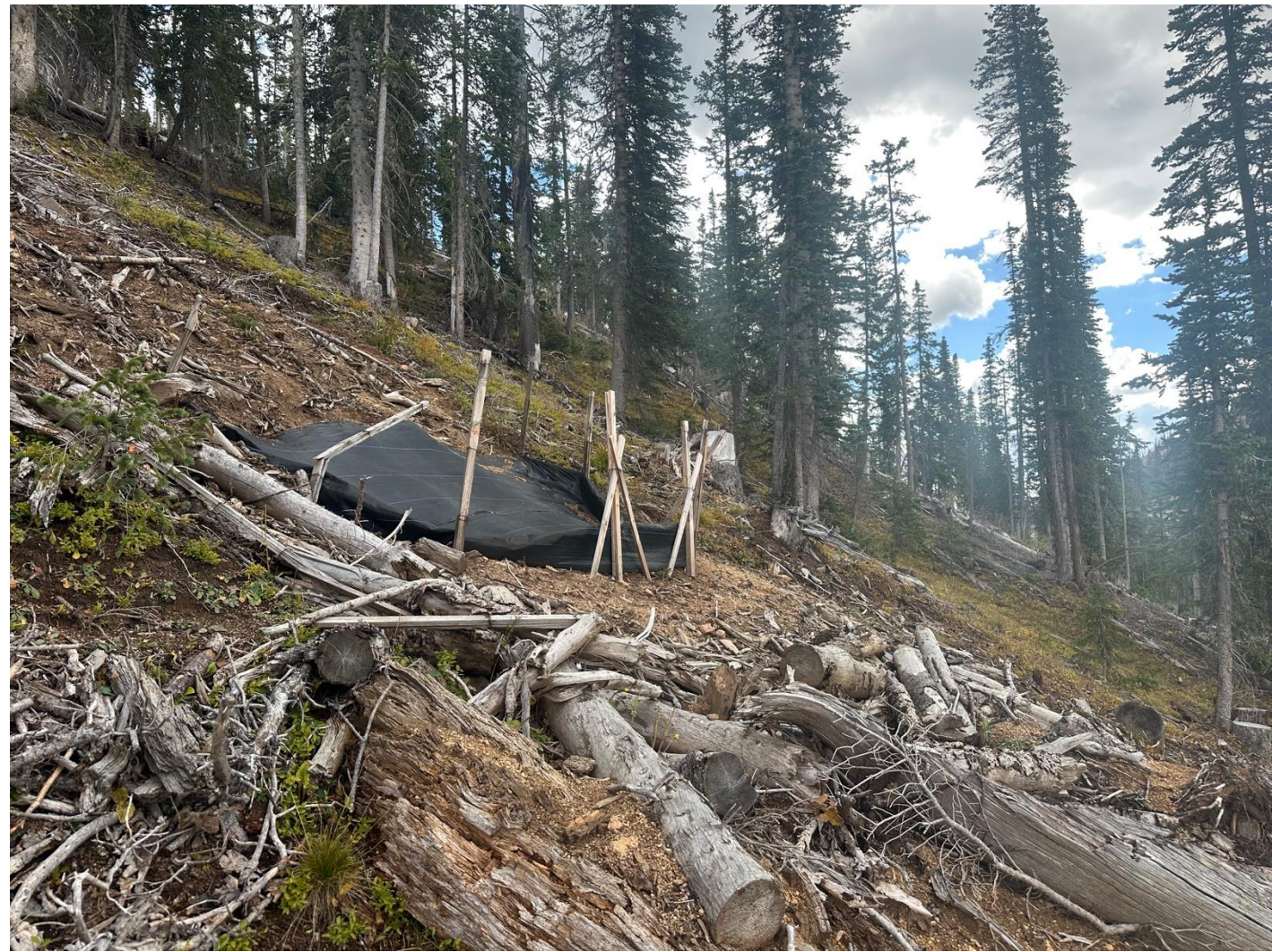
Another tarp and stake “mitigation” measure.
