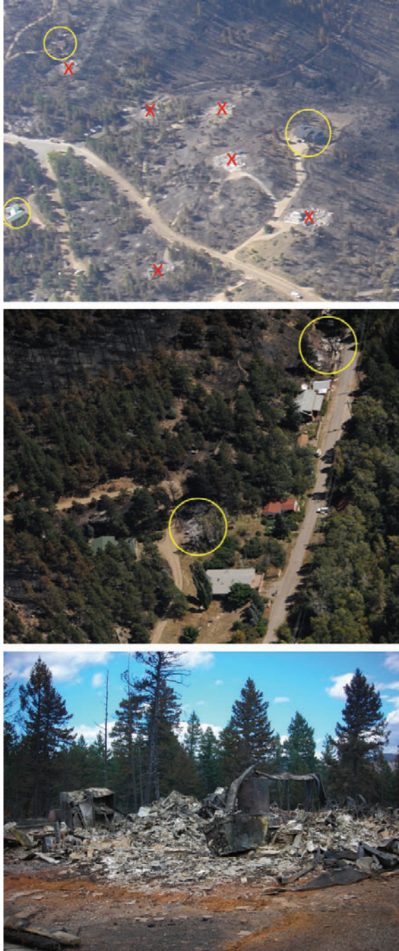
Figure 57. Top photo shows surviving homes (O) with destroyed neighbors (X) (photo: Dave Zader). The middle photo shows destroyed homes (O) with surviving neighbors (photo: Joe Amon). The bottom photo shows a destroyed home with adjacent green vegetation (photo: Boulder County Sherriff Office).
