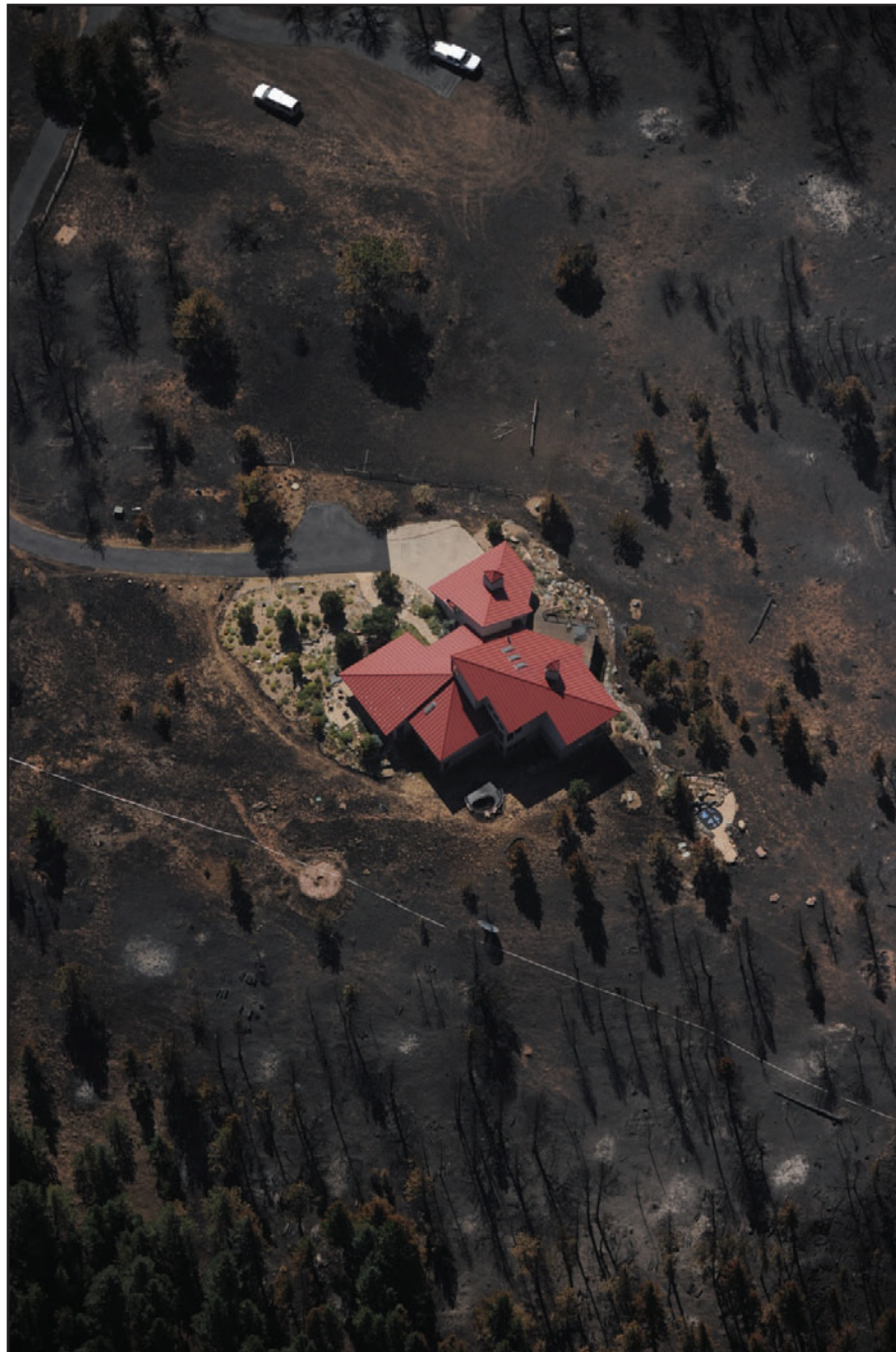
Figure 55. This is an example of a home ignition zone (HIZ) and how it reduces ignition potential within 100 feet of a home. Home construction was nonflammable or ignition resistant. Areas adjacent to the home were irrigated plantings or nonflammable materials. Firebrands landing on and around the home had few flammables to ignite. Surface fires were not eliminated within the HIZ but importantly, were restricted by the landscaping design from burning to contact the home. Trees that would produce high intensities were separated, thereby reducing the chances of canopy burning and, when not prevented, the burning canopies produced significantly less radiant heating to the home (photo: Joe Amon).
