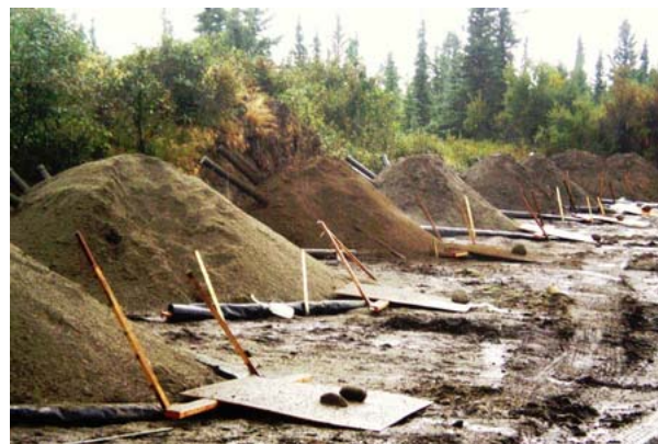
Figure 4. Soil berms with high amounts of soil organic matter and clay minerals as shown in this picture tend to retain concentrations of metal(loid)s as a result of large surface area and active binding sites. Image shows constructed shooting range berms in Delta Junction, Alaska on the Donnelly Training Area. Photo by A.J. Barker.
