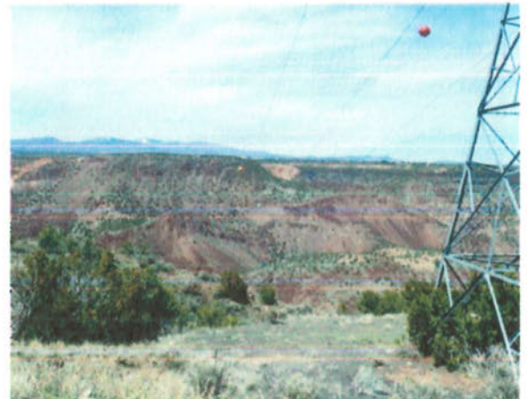
The existing electrical transmission line crossing the Rio Grande to LANL (called the Reeves Line). The proposed path forward would cross at the same location.
