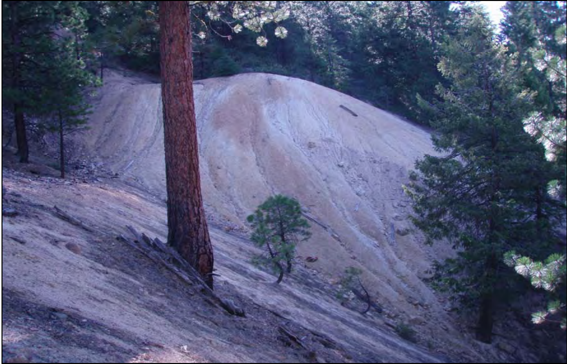
Photo No. 9: View of upper waste dumps showing signs of significant erosion (looking east).
