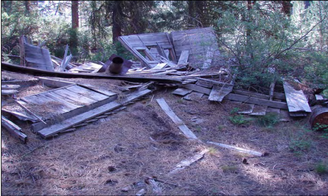
Photo No. 6: View of former lab sample structure below main road (looking east). SS3 was collected near the bottom of the picture.
