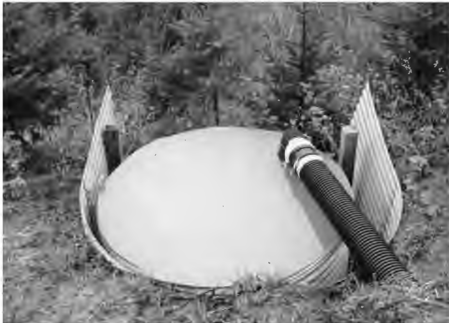
Figure 3. Photograph of sediment trap with crossdrain outlet.
