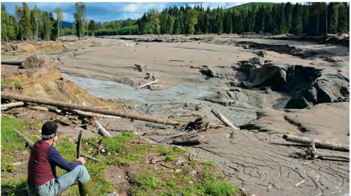
Fig. 2. Example of a catastrophic tailings dam failure. Tailings from the Polley Mine spill deposited over Hazeltime Creek ( https://watershedsentinel.ca/articles/mount-polley-mine-is-still-pumping-waste-into-quesnel-lake/ ). Before the spill, the creek was 5-m wide, with a cobble and gravel bed and forested riparian zone (Byrne et al., 2018).
