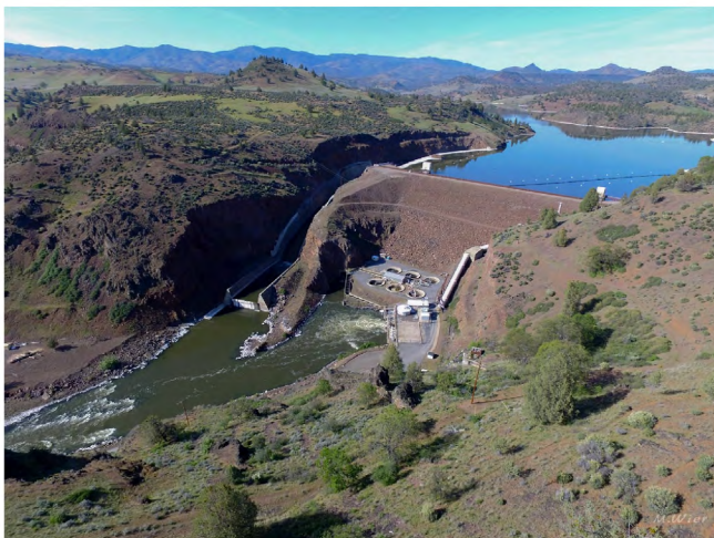
Fig. 6. Iron Gate Dam (53-m high, 226-m long; from Michael Wier, Klamath River Renewal Corporation).
