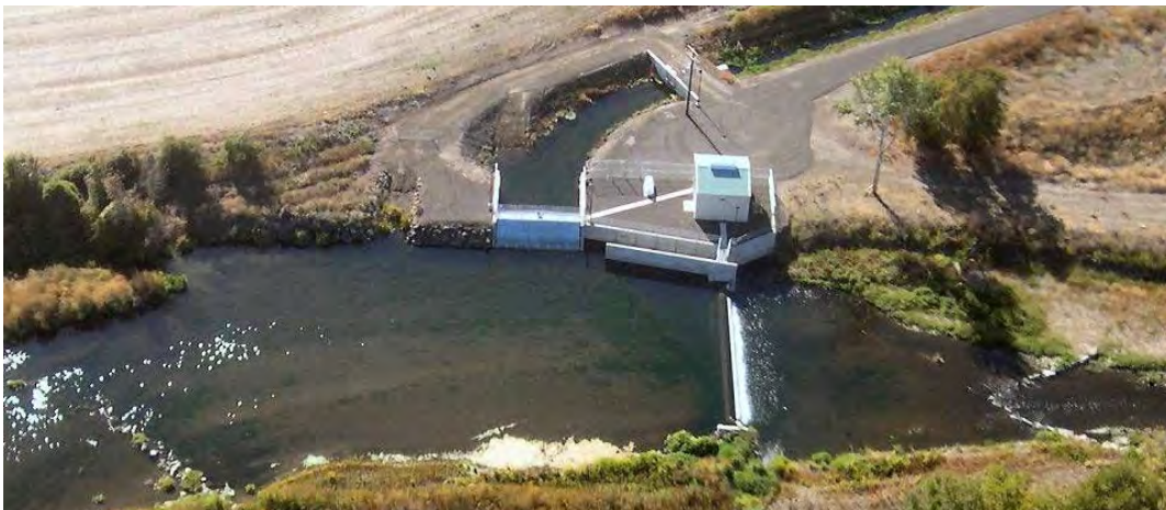
Figure 8-1. Aerial view of the Garden City-Lowden 2 water diversion on Walla Walla River near Touchet, Washington (Notes: River flow is from left to right. The bankline screen is located at the head end of the canal, just upstream of the spillway and adult ladder exit.)
