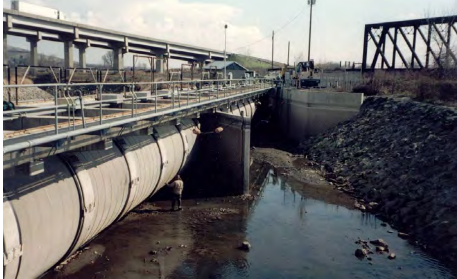
Figure 8-7 Large-sized rotary drum screen at the Sunnyside Canal located on the Yakima River near Yakima, Washington
