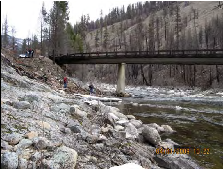
Figure 2. —West abutment, pier 1, and river bank.
