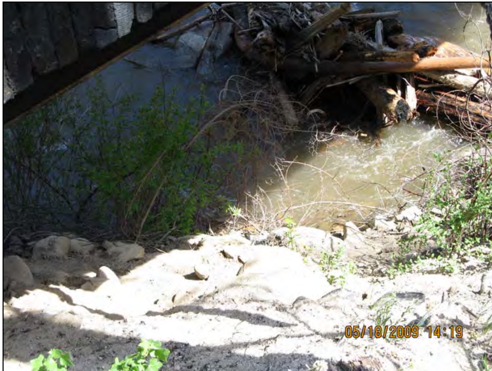
Figure 15. —Large woody debris accumulation at McCall side of EFSFSR bridge.
