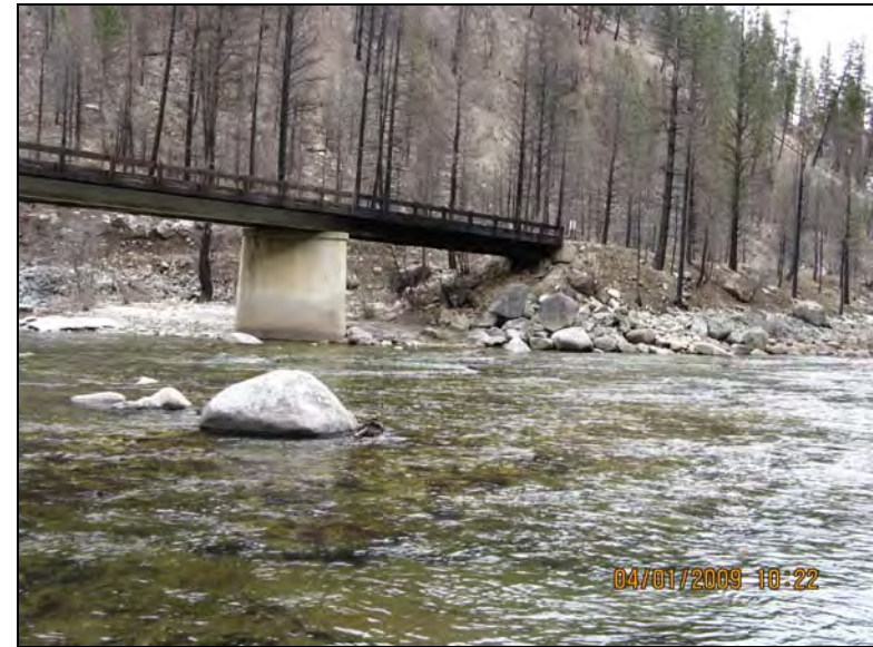
Figure 3. —East side abutment and pier 3.
