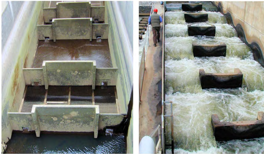
(a) Looking downstream
