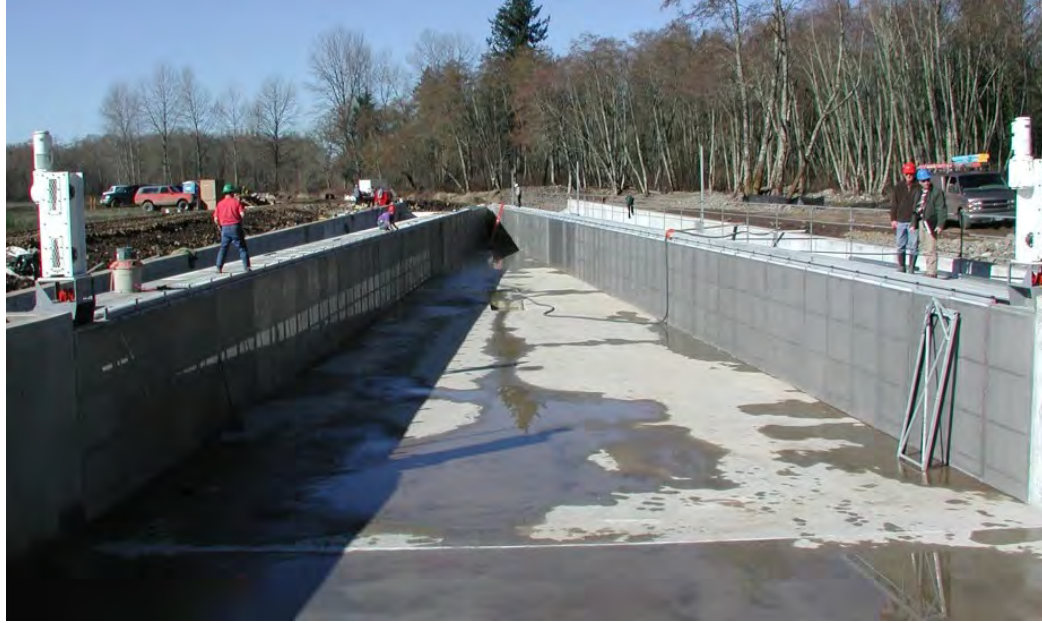
Figure 8-5 Vertical plate screen facility under construction in a diversion canal located on the Santiam River near Stayton, Oregon
