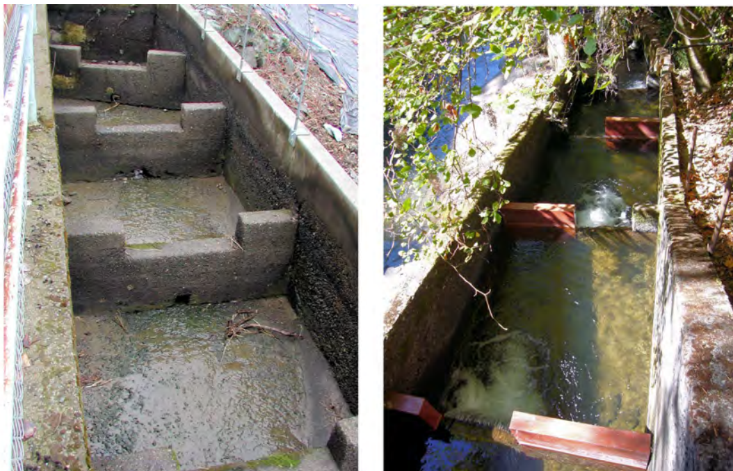
Figure 5-6. Examples of pool and weir ladders
