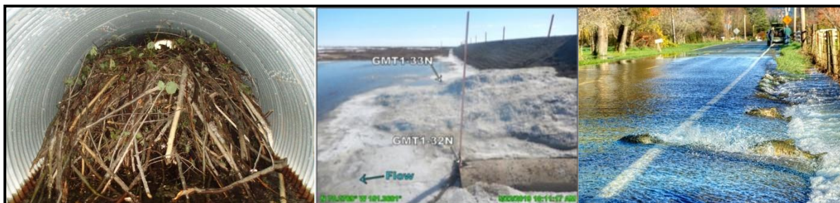
Figure 4. Examples of common causes of culvert blockages: beaver activity (left), ice on Alaska’s North Slope (middle), and flooding (right). Images from lizottesolutions.com, Michael Baker International 2019, and thurstontalk.com.
