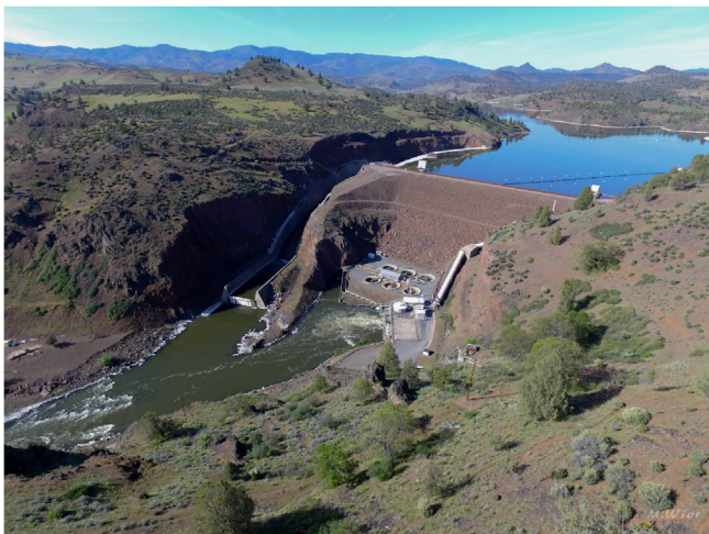
Fig. 6. Iron Gate Dam (53-m high, 226-m long; from Michael Wier, Klamath River Renewal Corporation).
