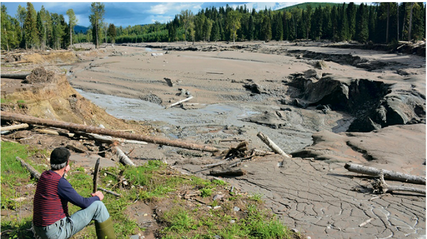
Fig. 2. Example of a catastrophic tailings dam failure. Tailings from the Polley Mine spill deposited over Hazeltime Creek ( https://watershedsentinel.ca/articles/mount-polley-mine-is-still-pumping-waste-into-quesnel-lake/ ). Before the spill, the creek was 5-m wide, with a cobble and gravel bed and forested riparian zone (Byrne et al., 2018).
