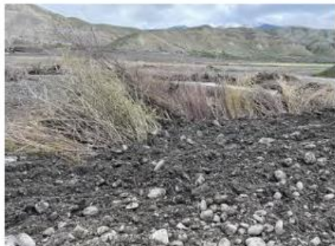
STAGE 3: TRENCH BACKFILLED WITH NATIVE ALLUVIUM AND ORGANIC TOP LAYER BEING PLACED.
