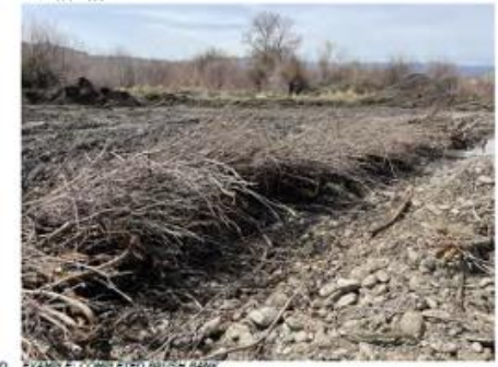
STAGE 1: MUD SLURRY IN BOTTOM OF EXCAVATED TRENCH WITH LIVE CUTTINGS PLACED. EXAMPLE: COMPLETED BRUSH BANK.
