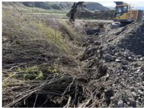
STAGE 2: VERTICAL SLASH/RACKING PLACED AND BACKFILLING TRENCH WITH NATIVE ALLUVIUM.
