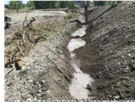
STAGE 1: MUD SLURRY IN BOTTOM OF EXCAVATED TRENCH WITH LIVE CUTTINGS PLACED. EXAMPLE: COMPLETED BRUSH BANK.
