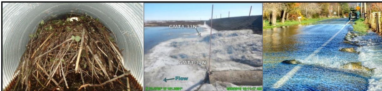
Figure 4. Examples of common causes of culvert blockages: beaver activity (left), ice on Alaska’s North Slope (middle), and flooding (right). Images from lizottesolutions.com, Michael Baker International 2019, and thurstontalk.com.
