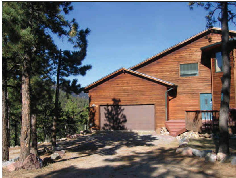
Figure 13. A total of 474 homes were located in the area where the Fourmile Canyon Fire burned (photos: Russ Graham).
