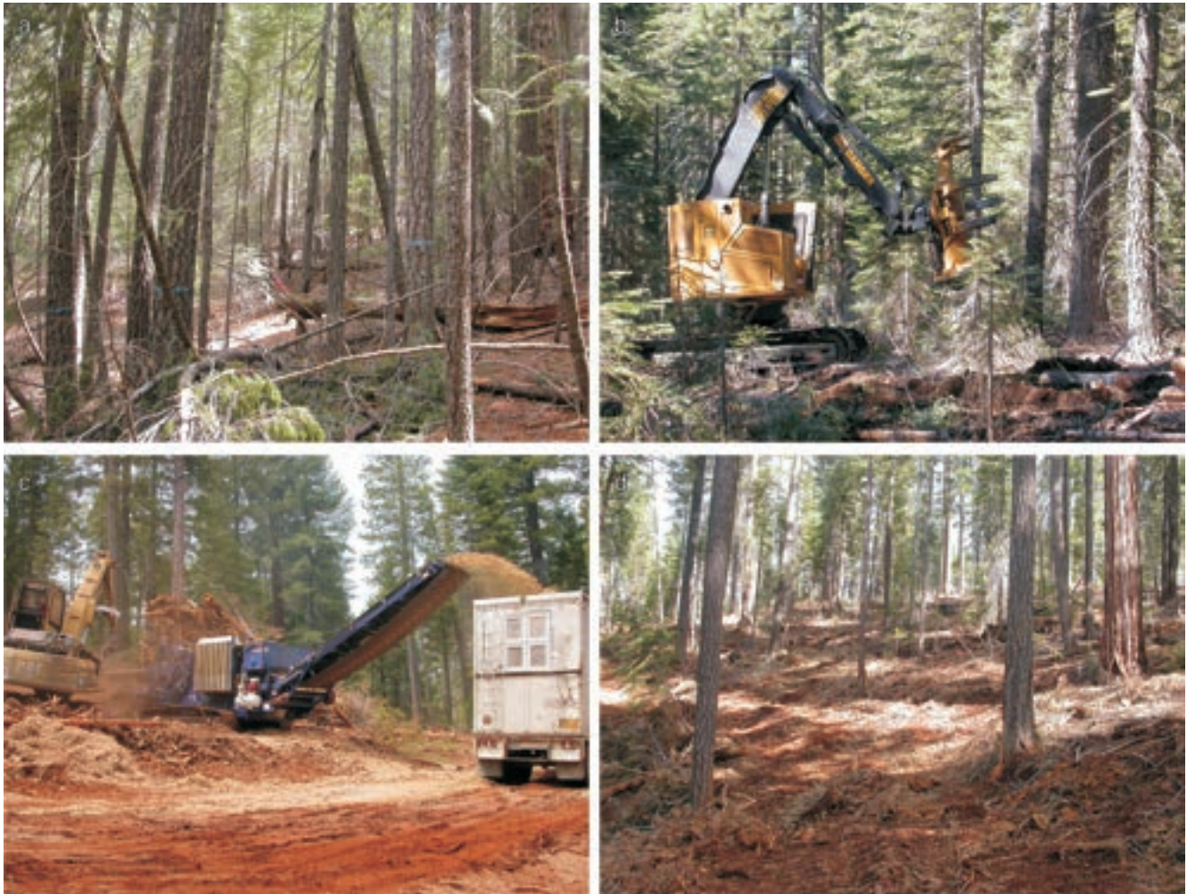
Figure 1. Fuel treatments implemented in the Meadow Valley project area. (a) Pretreatment mixed-conifer forest. (b) Whole-tree harvester cutting small trees (thinning from below). (c) Small trees, tree tops, and limbs being chipped and shipped by truck to a bioenergy plant to produce electricity. (d) Posttreatment defensible fuel profile zone, taken from the same perspective as in panel (a). Photographs: Keith Perchemlides.
