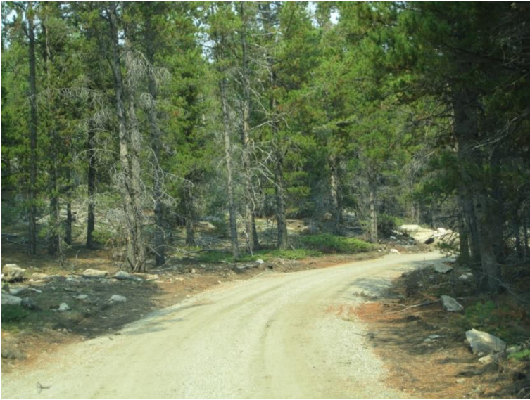
6 Forest Road 382 after undisclosed upgrades completed.
