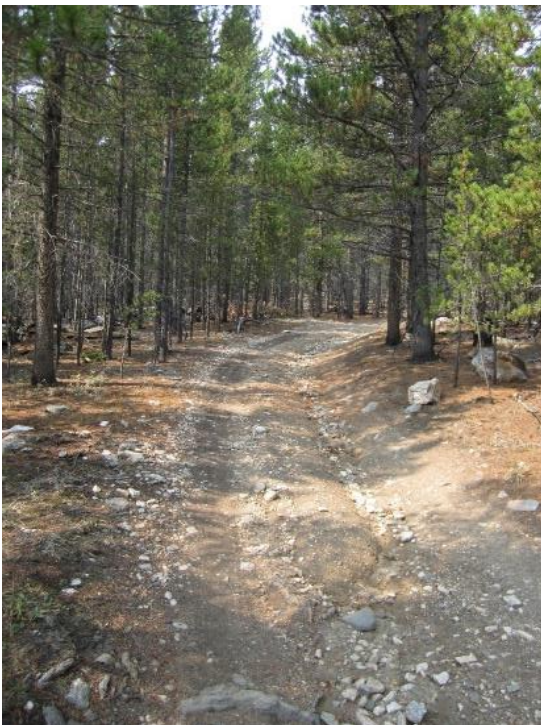
5 Forest Road 382 prior to upgrading activity for the BMW project.
