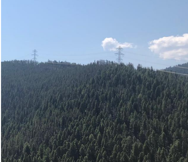
Powerline in Project area under dense fuels.
