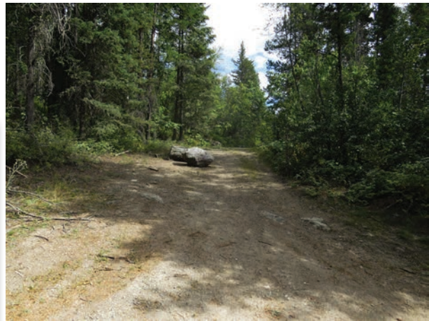
Fig. 8: 8/25/16 view of closed road 5392Y from road 5392.
