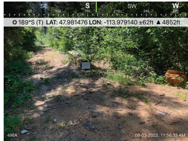
Fig. 17: Berm driven over by pickups on road 498A.
