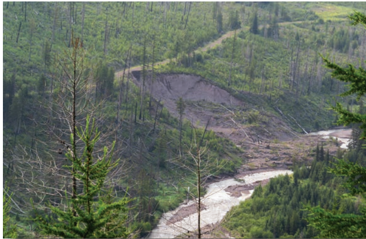
Water collecting in the ditch of this closed road contributed to mass failure into Sullivan Creek, a key bull trout spawning stream.
