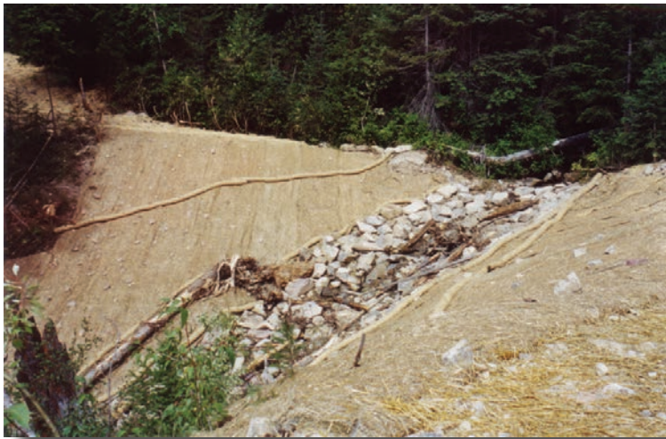
Road decommissioning removes culverts, restores streambed gradients, removes road fill, and stabilizes slopes. Paul Harvey photo
