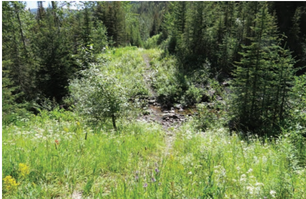
The last three miles of Bunker Creek Road 549 was decommissioned under Clinton's 1998 Clean Water Action Plan. Here a bridge was removed at Warrior Creek.
