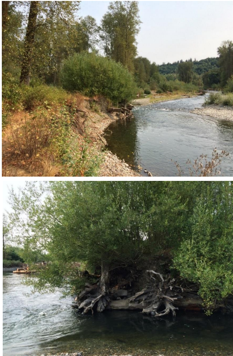
Figure 2. Engineered log jams stand out when first installed but become integrated into the landscape as vegetation develops. This ELJ on the Cedar River in King County was installed in fall 2010 (Lorin Reinelt, King County engineer, personal communication). Above: View upstream. Below: close-up of ELJ components: anchor posts, cribbing logs, rootwad logs, rock ballast and gravel fill. Willow has fully colonized this ELJ. Photos by Jim Evans, September 4, 2017.
