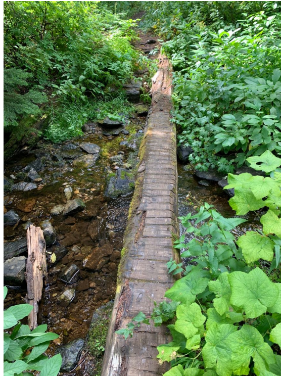
Log bridge on the Oregon Lakes Trail.
