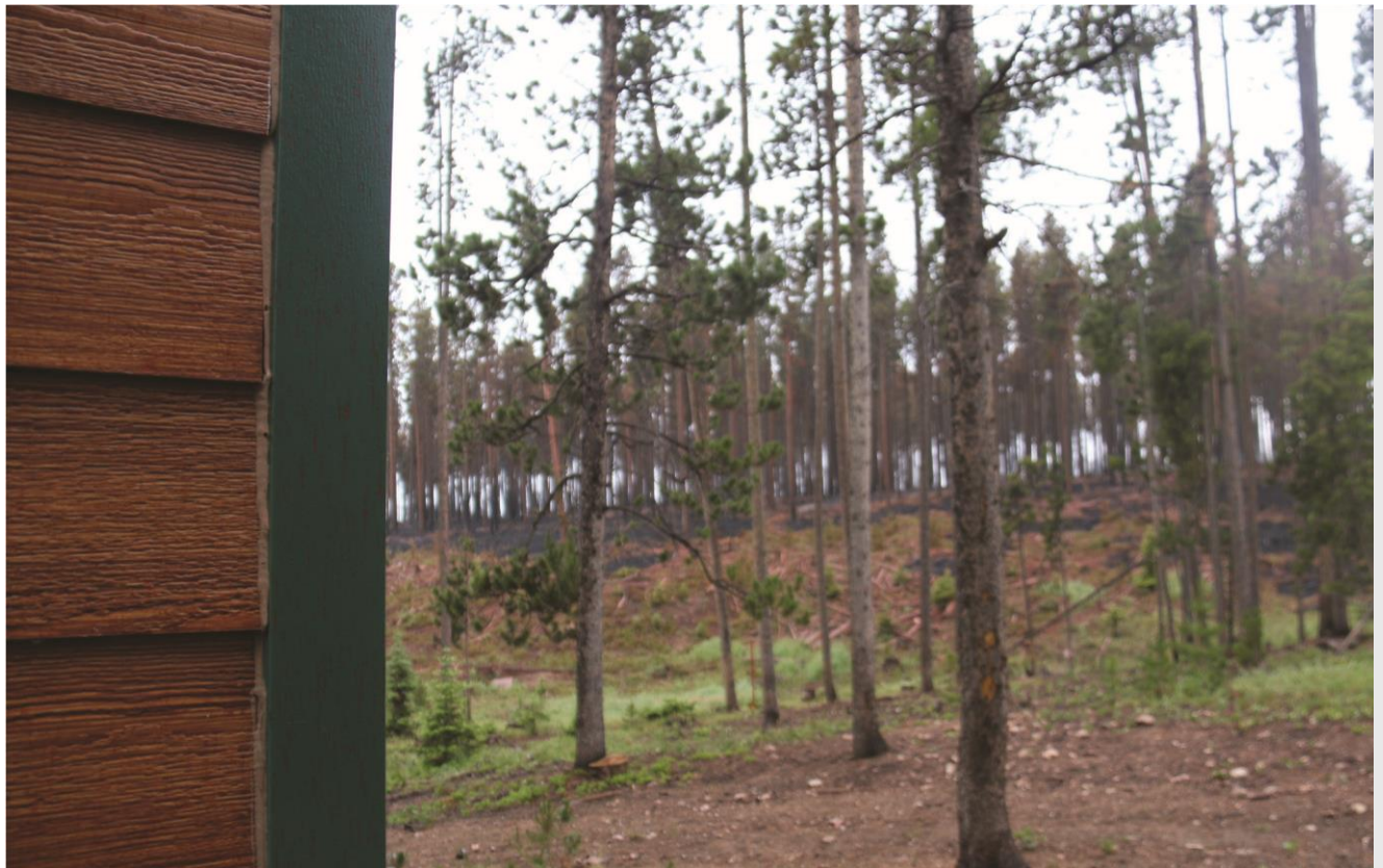
Defensible space around a home reduced the fire’s intensity as it neared the property.
