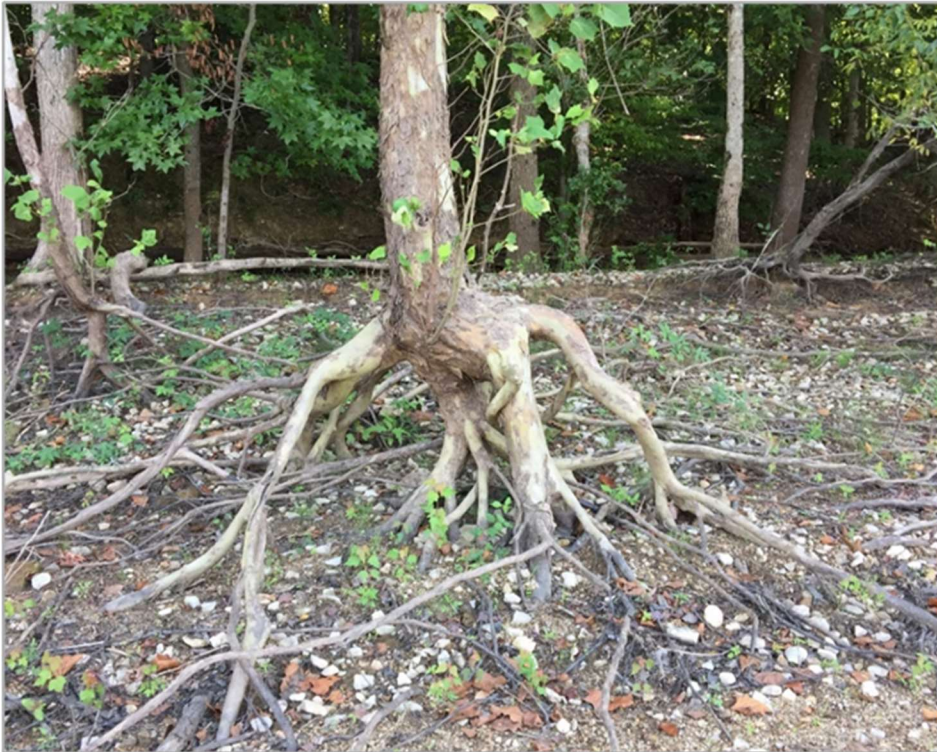
Figure 10: Bare Roots Show the Extent of Monroe Lake Shoreline Erosion
