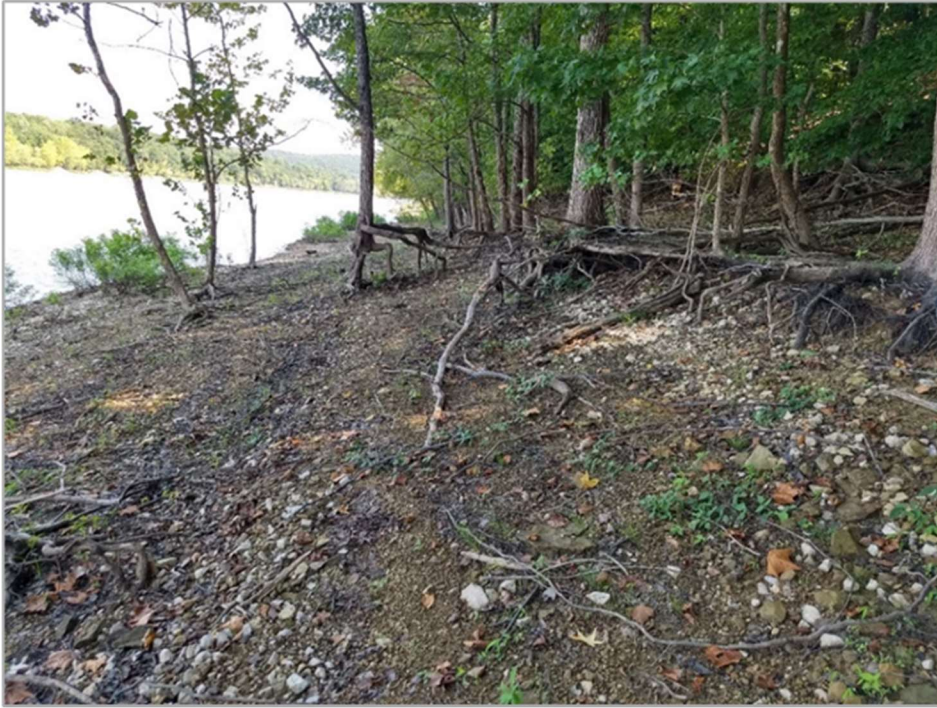
Figure 9: Monroe Lake Shoreline Erosion
