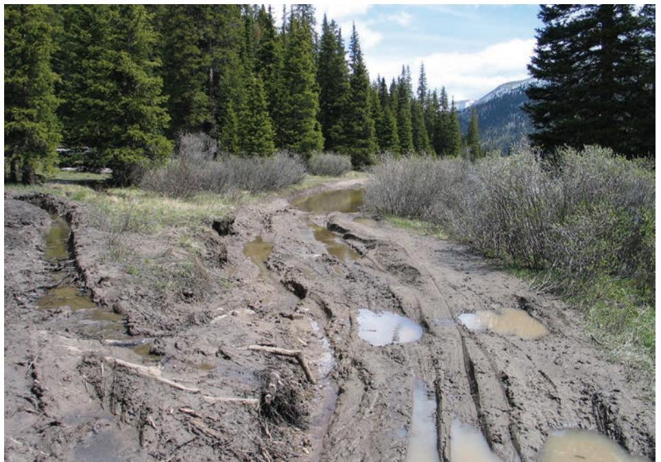
Top: A road blow-out on the Mt. Baker-Snoqualmie National Forest. Bottom: Poor drainage and maintenance is resulting in erosion, habitat damage, and public access challenges on the Arapahoe National Forest.
