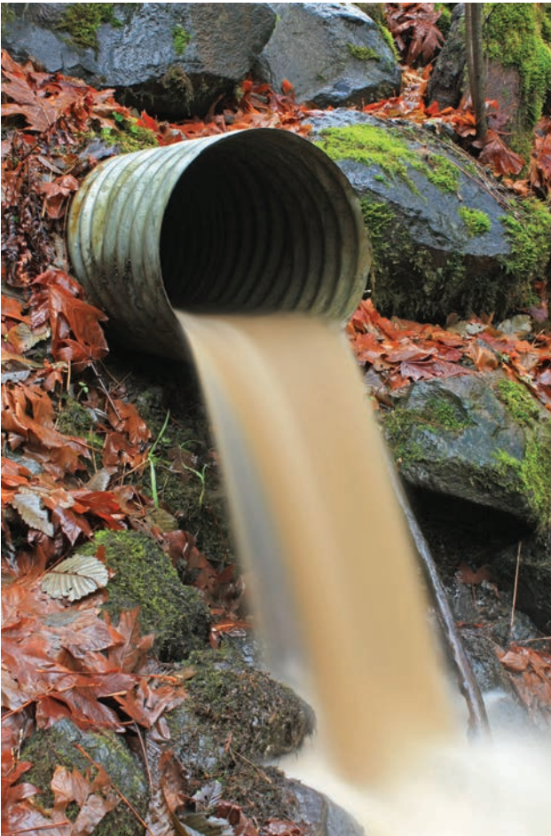
Top: Inadequate road design or maintenance can lead to enormous erosion and the dumping of sediment into streams and rivers.
