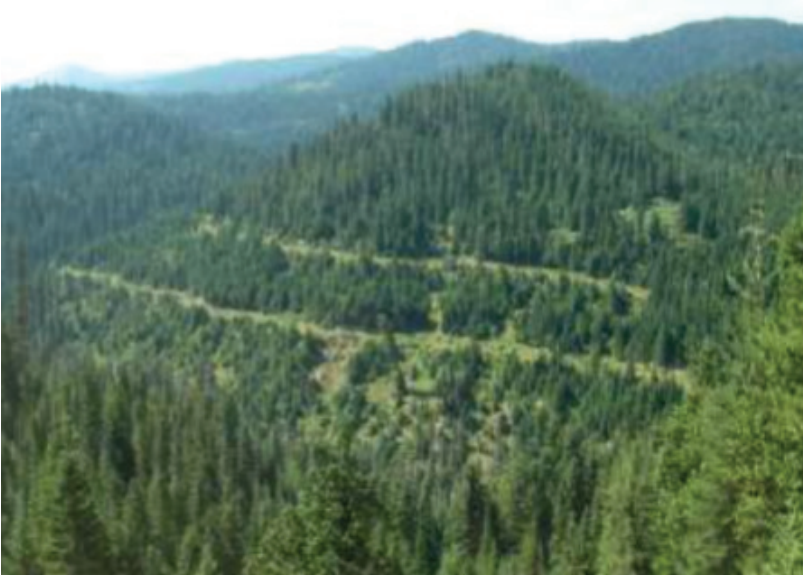
Collapsing roads on the Clearwater National Forest.
