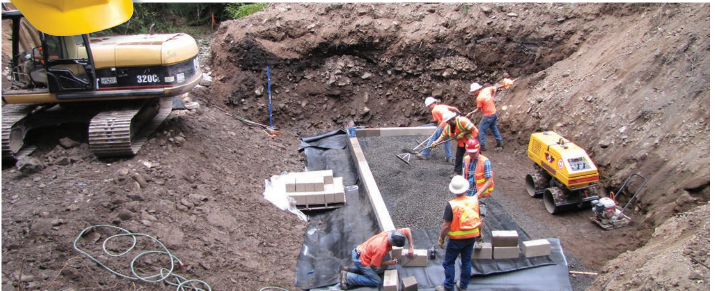
Culvert to bridge construction, Gifford Pinchot National Forest.
