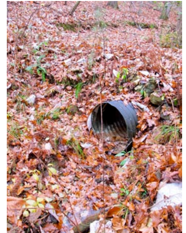
Installed above substrate
