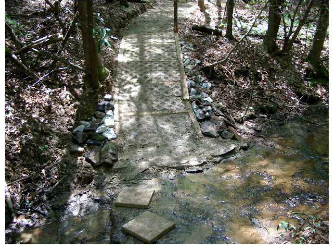
Full box turfstone armoring, beginning from stream gradient and continuing upslope
