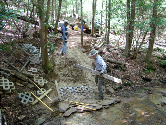
Full box turfstone armoring, beginning from stream gradient and continuing upslope
