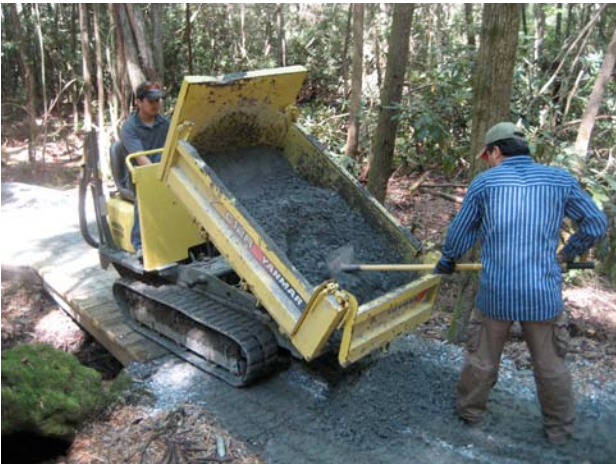
Trail hardening application near stream crossing to prevent sedimentation
