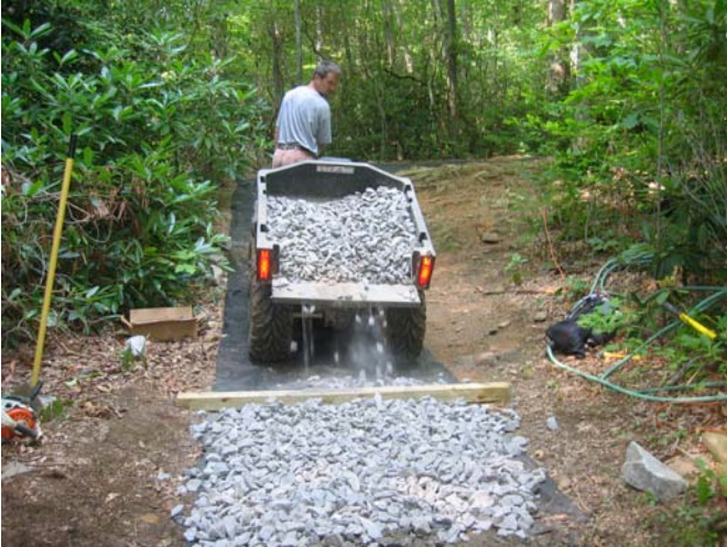
Raised tread hardening application with railroad ballast (and intermittent lateral rock migration additions) topped by crushed and compacted limestone
