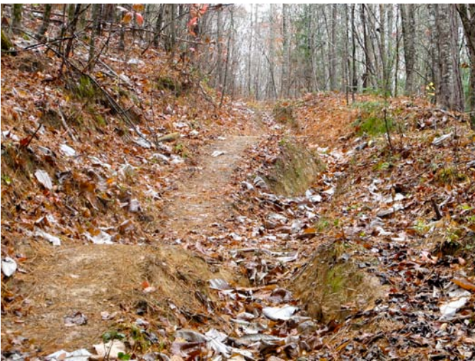
Old forest road (proposed for trail system) with failed water management
