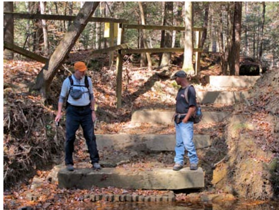
Upper Brushy Creek crossing structure- very steep stream entrance, scour beginning at base
