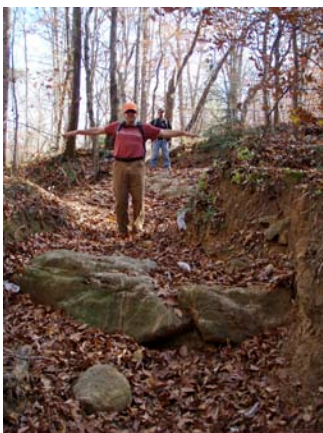
Trail incision to bedrock. No trail grade in these photos is greater than 20%
