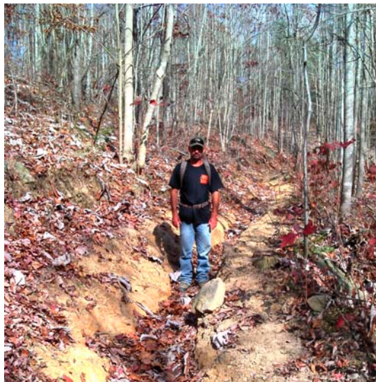
Steep, severely eroded trail sections where maintenance has a very low probability of success. Relocation necessary.
