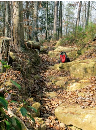
Steep, severely eroded trail sections where maintenance has a very low probability of success. Relocation necessary.
