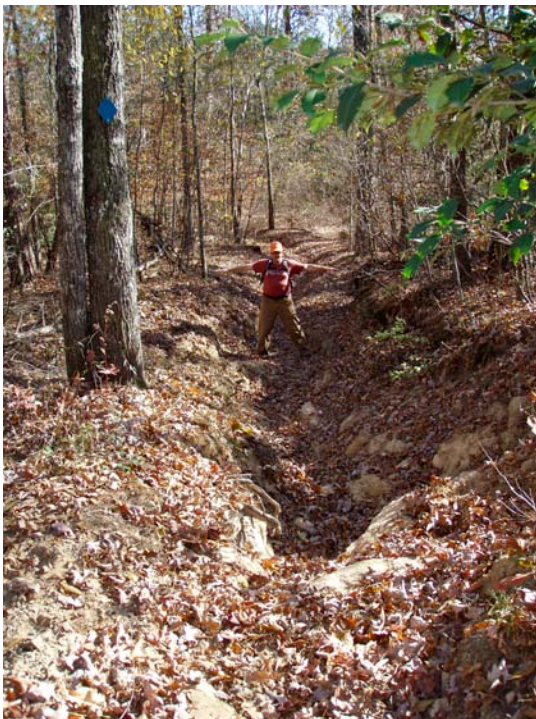
20% gradient trail, incised to a depth of 5'
