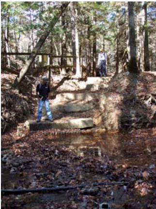
Upper Brushy Creek crossing structure- very steep stream entrance, scour beginning at base
