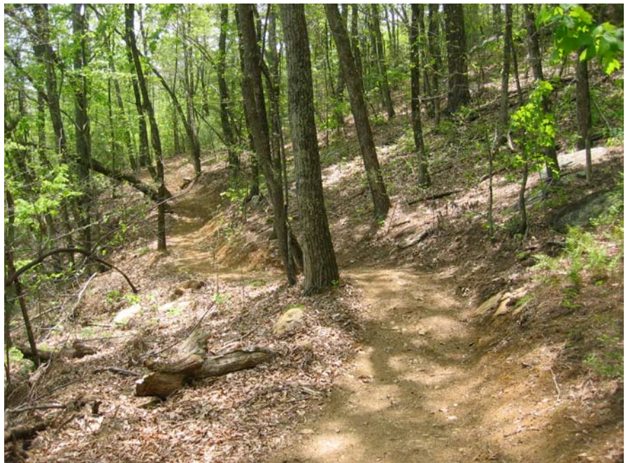
Lack of rolling contour design results in lengthy erosion sections. Rolling grade designed into relict forest management route and relocations will better control the flow of water and sediment.
