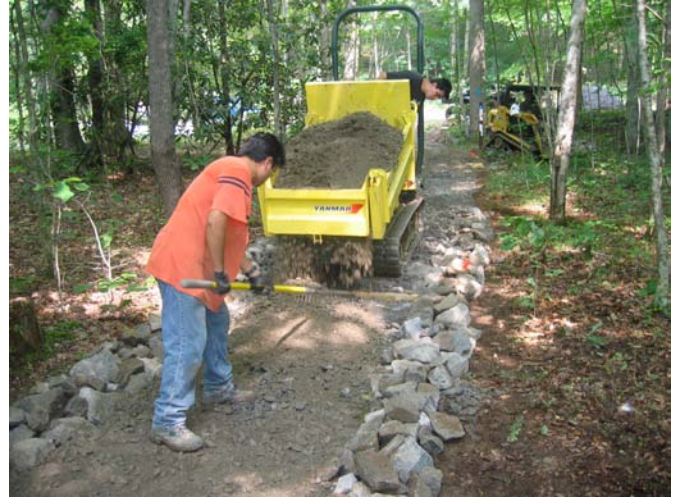
Raised tread hardening application with railroad ballast (and intermittent lateral rock migration additions) topped by crushed and compacted limestone
