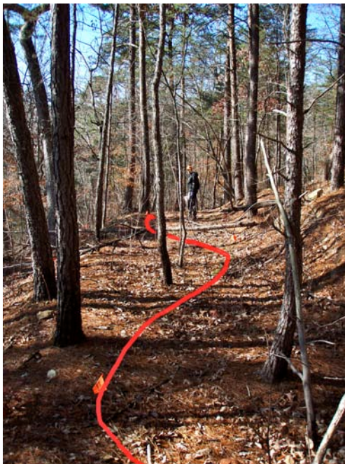
Lack of rolling contour design results in lengthy erosion sections. Rolling grade designed into relict forest management route and relocations will better control the flow of water and sediment.
