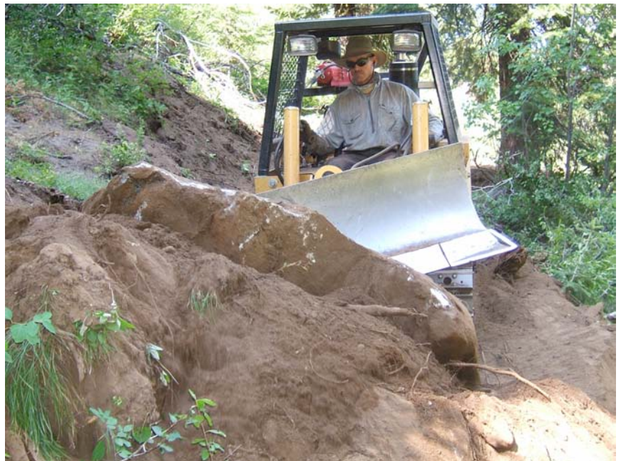
Powerful Sweco 480 Trail Dozer moving large rock and soil. The machine's power, combined with the sandy soils in Bankhead, hold the potential for causing as much trail damage as maintenance
