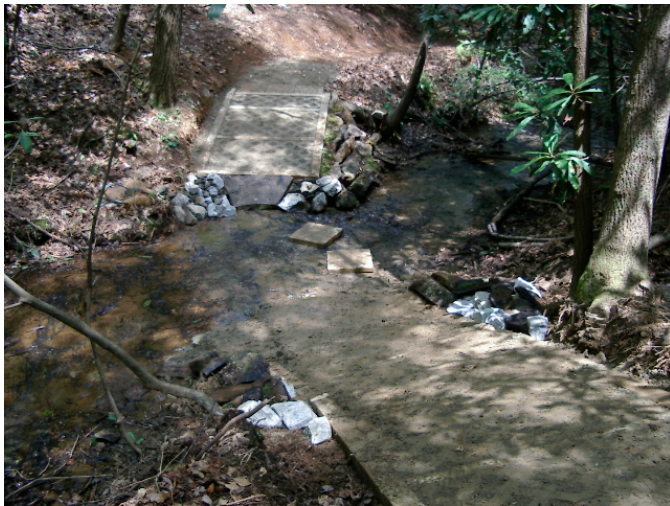
Finished project with rip rap flow protection and 7 years/1,000's of horse passes later
