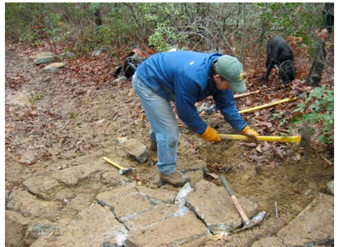
Broken concrete full box armoring in process and just prior to final joint fill
