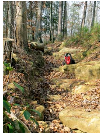
Trail incision to bedrock. No trail grade in these photos is greater than 20%
