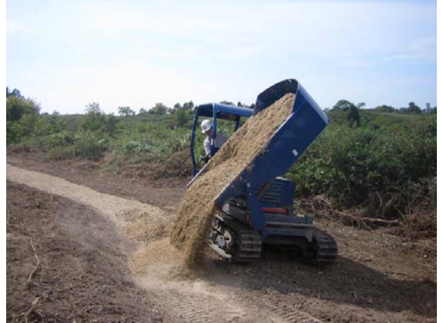
Minor excavation, then fill-to-grade in sandy soil to harden tread
