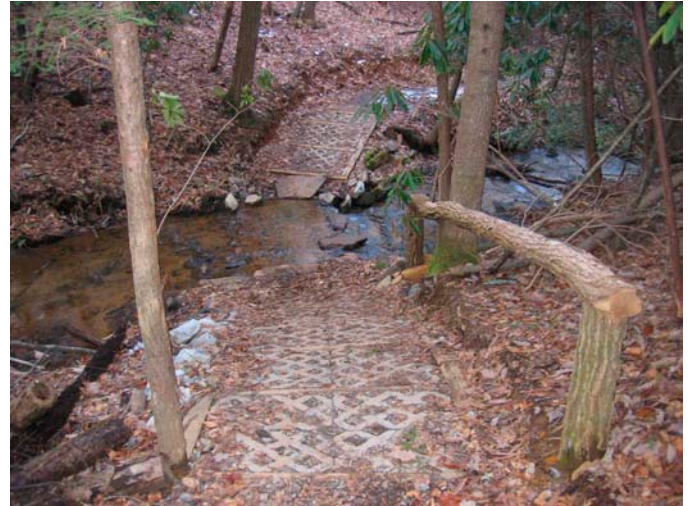
Finished project with rip rap flow protection and 7 years/1,000's of horse passes later
