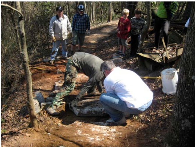
Broken concrete full box armoring in process and just prior to final joint fill
