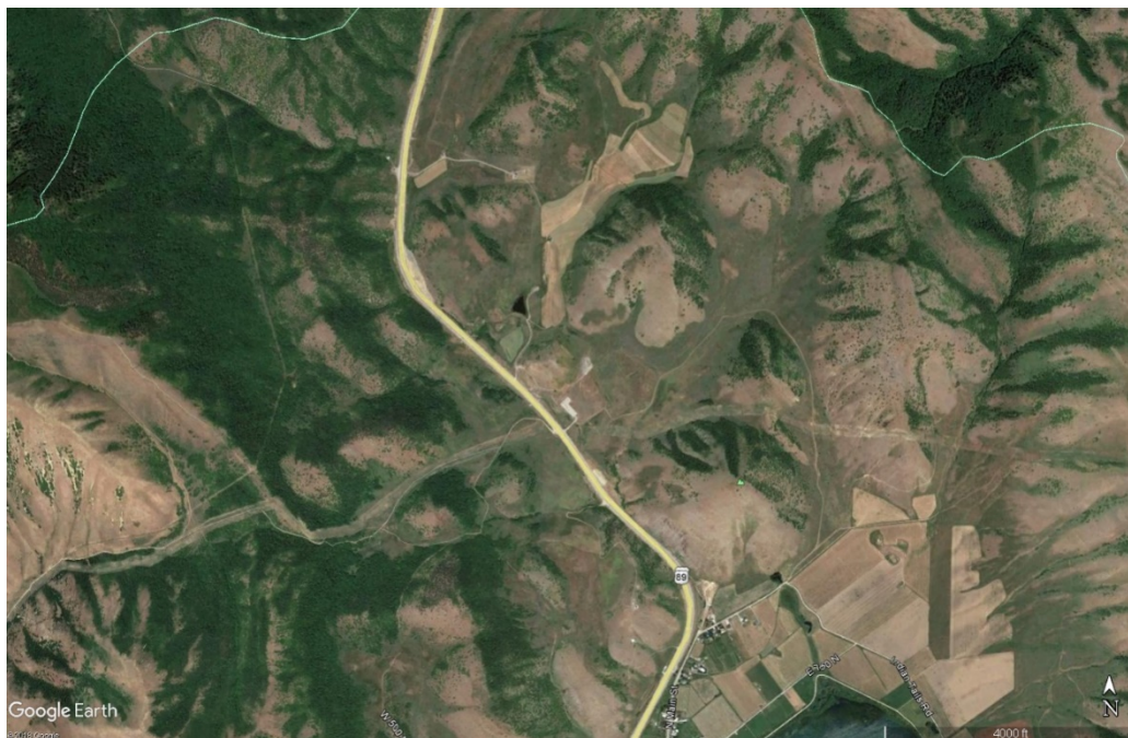
Figure 2. Ruby Pipeline near Mantua, Utah at about six years
