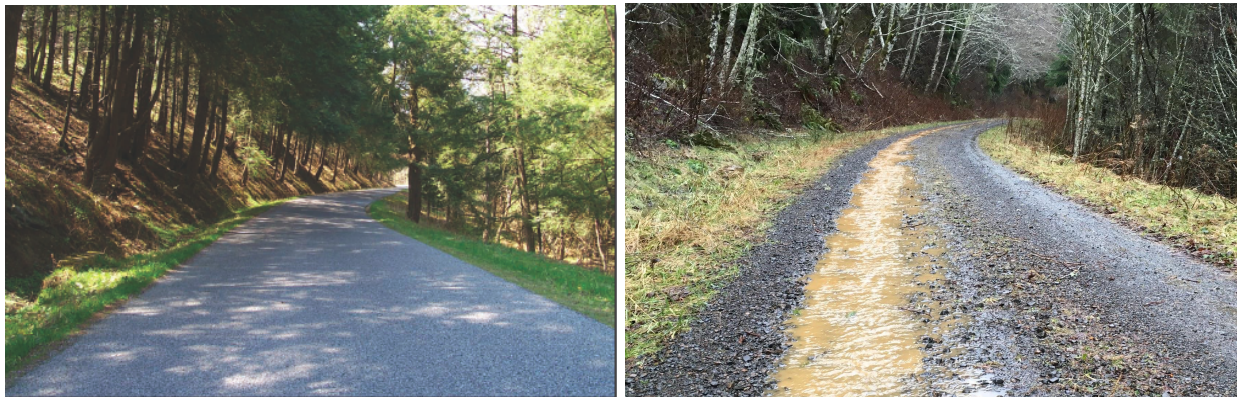
Figure 2. The photo on the left illustrates a typical “passenger vehicle” maintained road often with paved surface, wider road footprint, safety features such as guardrails and higher maintenance costs. The photo on the right illustrates a typical “high-clearance” vehicle road that is often natural surface, narrow road footprint, less maintenance costs which leads to gullies, ruts and potholes. As of 2018, 83% of national forest roads are minimally maintained in the “high-clearance” category.
